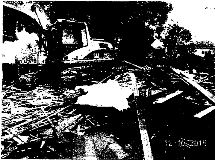
Demolition 2108 West 25 th Street December 10, 2015
