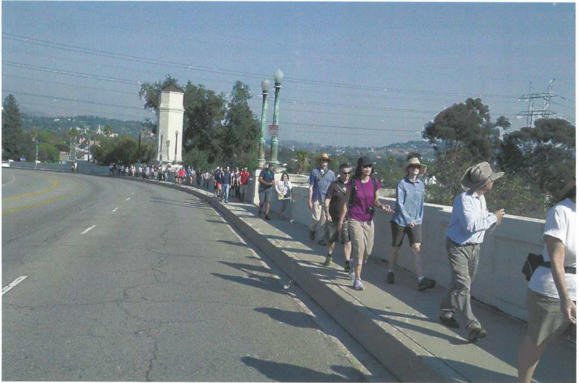
Photo of Hyperion Bridge South sidewalk looking north
