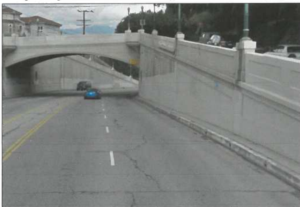
Figure 1. Sight Distance on Northbound Hyperion Avenue at Waverly Drive
