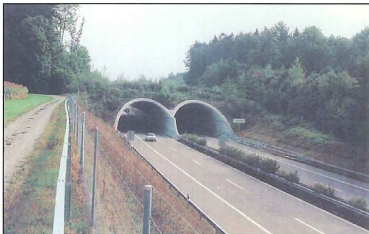
Design accommodates habitat, wildlife passage, trails, and vehicles Source: Scott Jackson, UDOT/FHWA 2000, p. 5.
