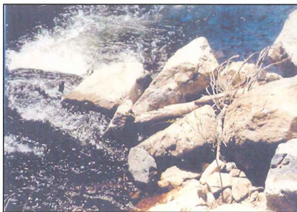
Rock spurs stabilize banks, aerate water, and make fish passage easier (Provo River, Utah, Utah DOT) Source: , UDOT/FHWA (Undated), p. 46.
