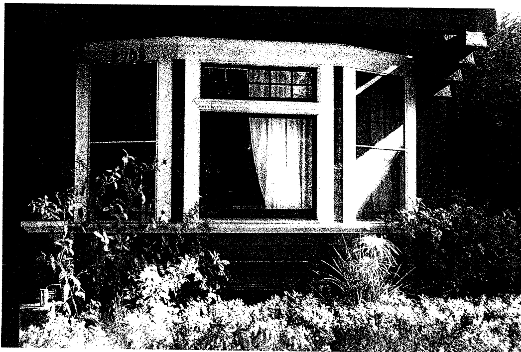
West façade detail: West slant bay paired nine-over one casement windows flank central fixed pane topped by ten light fixed transom, viewed to east.
