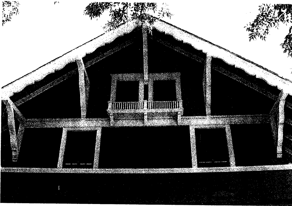
West façade detail: Corbel eave and bracket supports, shaped bargeboard, paired windows in gable end with bracket supported balcony with rail, full length overhanging balcony at second level with two pairs multi-paned French doors, viewed to east.
