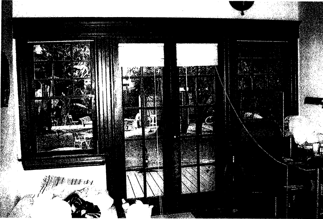
Library east wall: Original nine-over-one sash windows and added 10-light paired French doors opening unto rear deck and east lawn, viewed to east.
