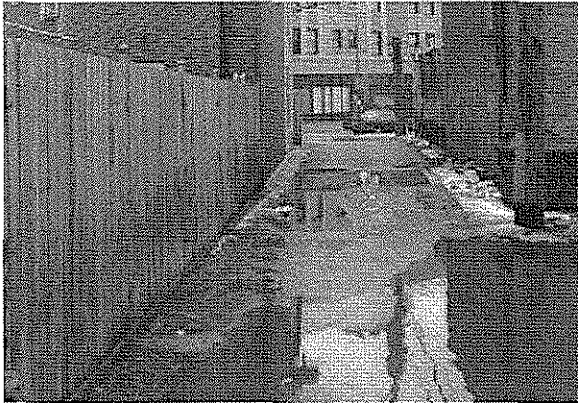
Figure 5. Chicago alley with impermeable pavement and poor drainage.
