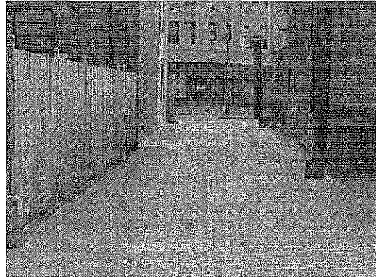
Figure 6. Chicago alley retrofitted with permeable pavement.
