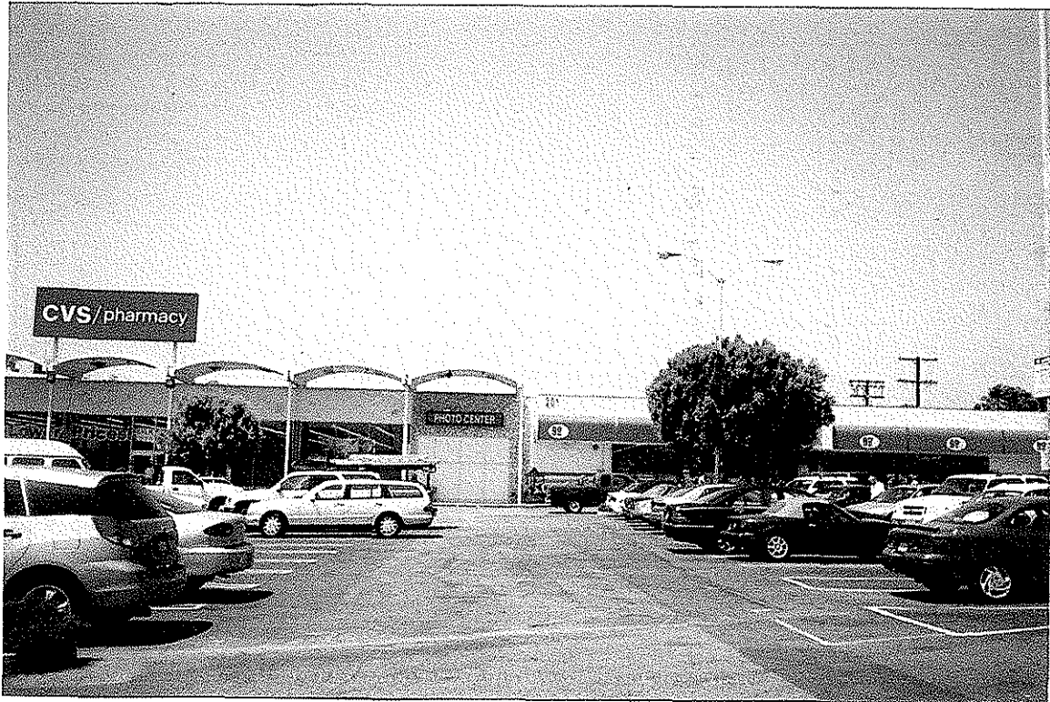
4. View of tenant space looking westerly from parking lot.
