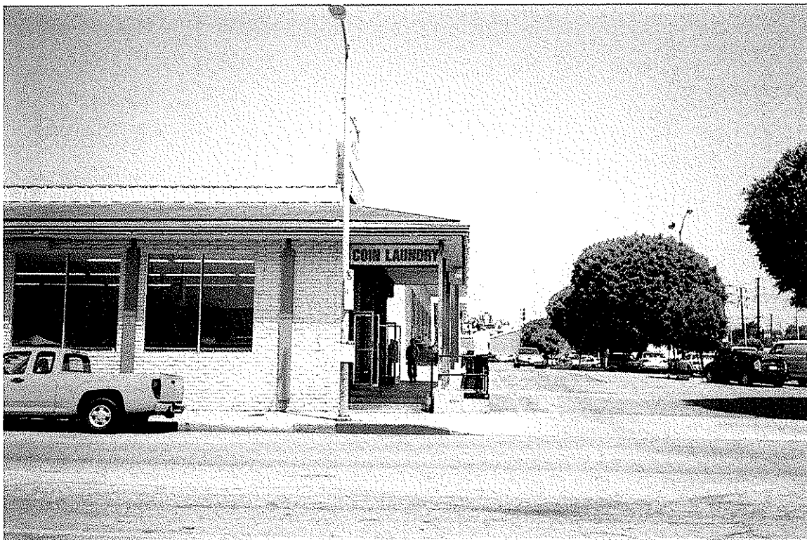
6. View of frontage looking northerly from Rose Avenue.
