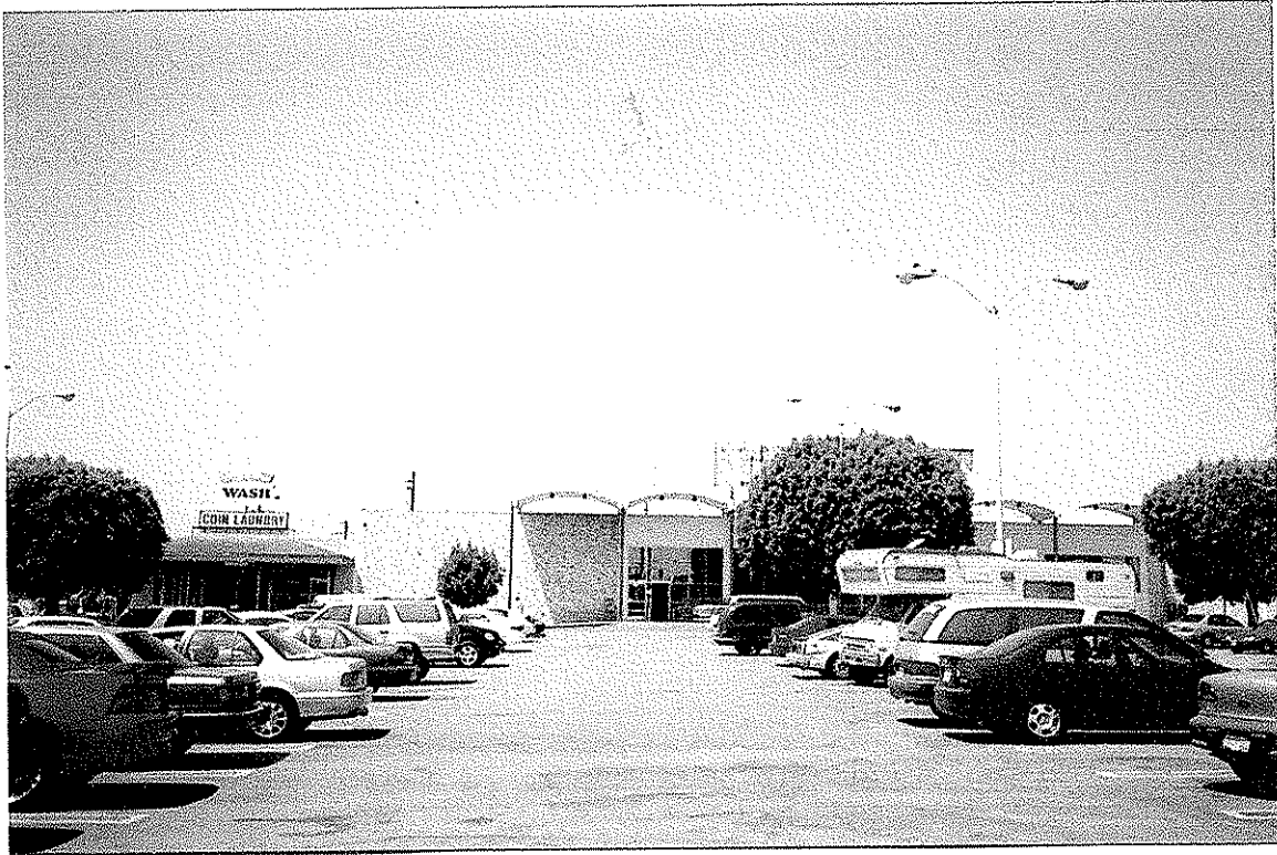
1. View of tenant space looking westerly from parking lot.
