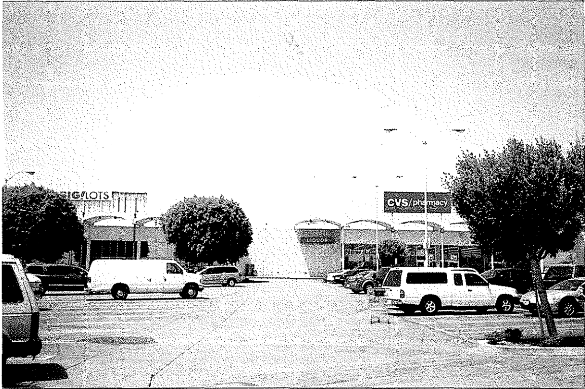
3. View of tenant space looking westerly from parking lot.
