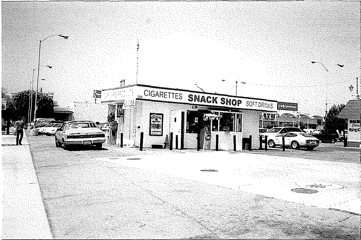
13. View of service station at SWC of Rose Avenue and Lincoln Boulevard.
