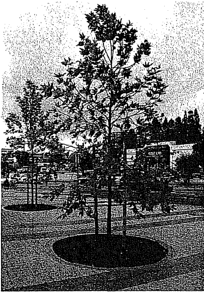
Tree with large tree well surrounded by permeable paving with gap graded soil to store and infiltrate stormwater beneath.
