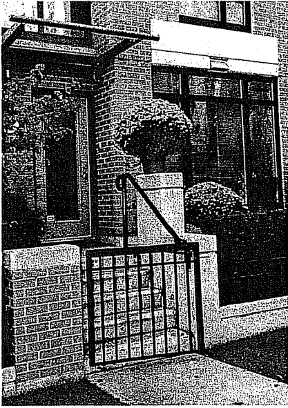
Good example of individual unit entry several feet above the sidewalk with porch and windows that look onto the street.
