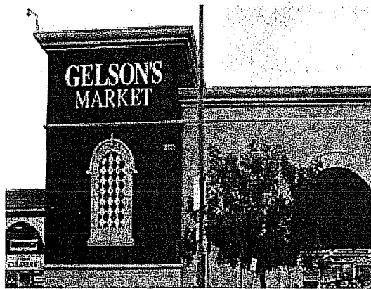
Signage well placed on building.
