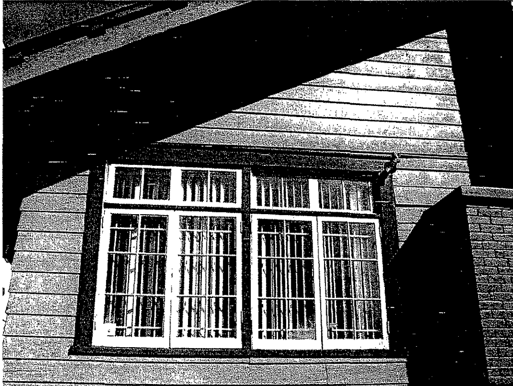
Original Echo Park Clubhouse, front casement windows, 1004 Echo Park Avenue (Photograph by Charles J. Fisher)
