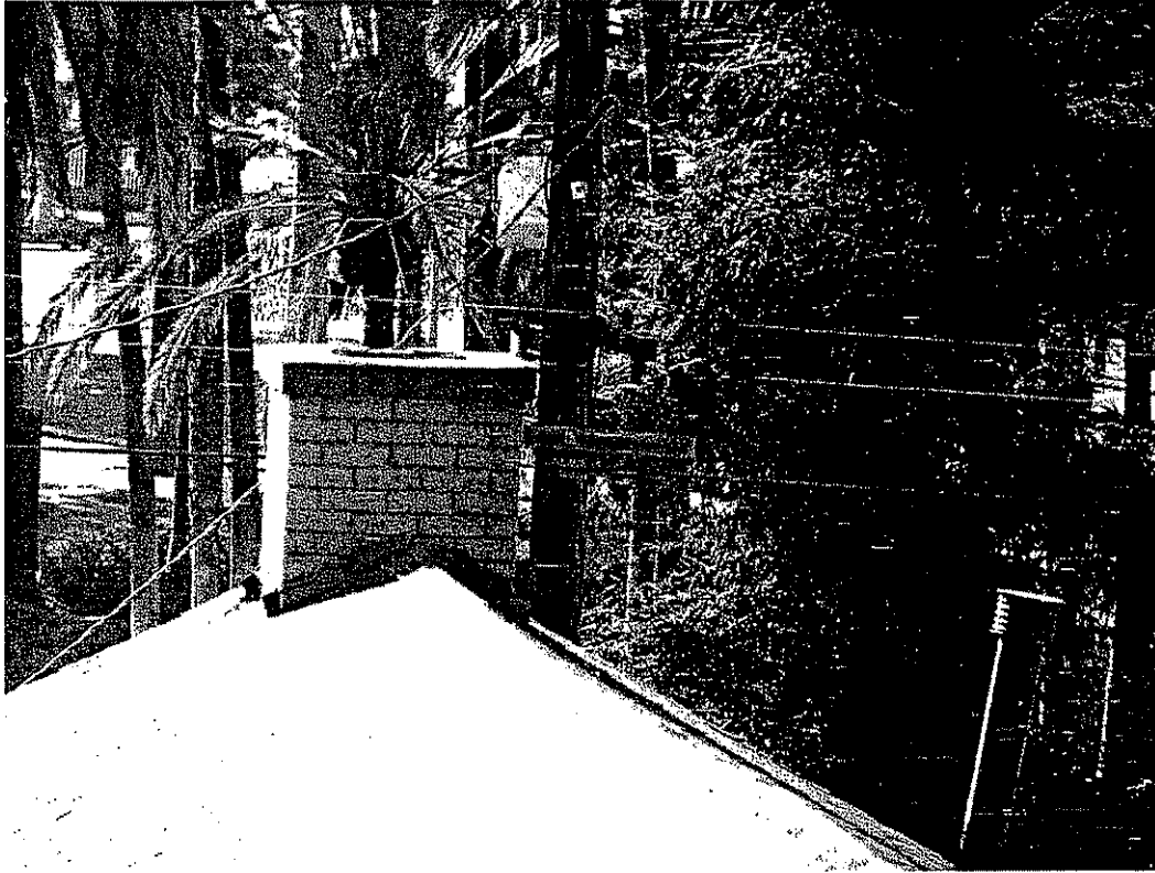
Original Echo Park Clubhouse, front chimney, 1004 Echo Park Avenue (Photograph by Charles J. Fisher)
