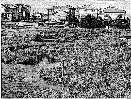
Regional stormwater detention facilities were used effectively to control runoff from new development in the Cherry Creek area.
