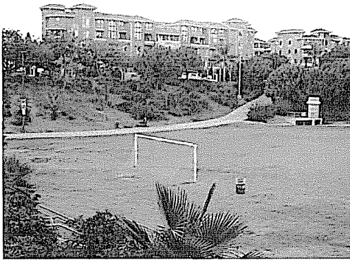
Pan Pacific Park in Los Angeles serves as both a recreational area and a stormwater treatment basin.
