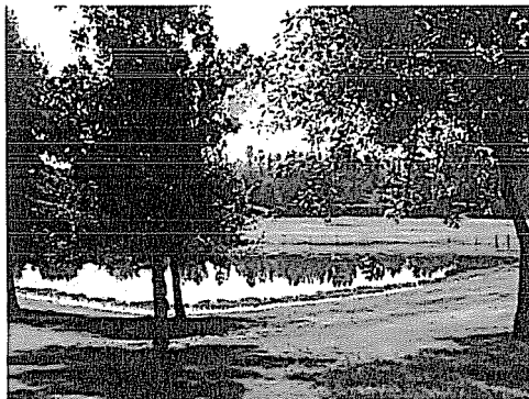
Detention and infiltration basins are used extensively in Fresno, Calif., for regional treatment of stormwater runoff.
