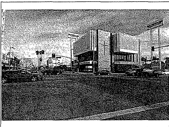
East view on Wilshire, 2008. (Underhill)
