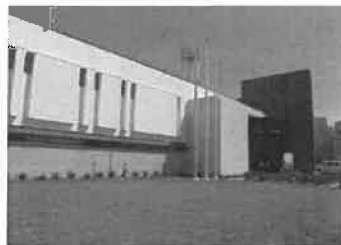
Rampart Area Replacement Station
