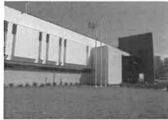
Rampart Area Replacement Station
