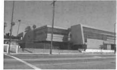
Olympic/20 th Area New Station
