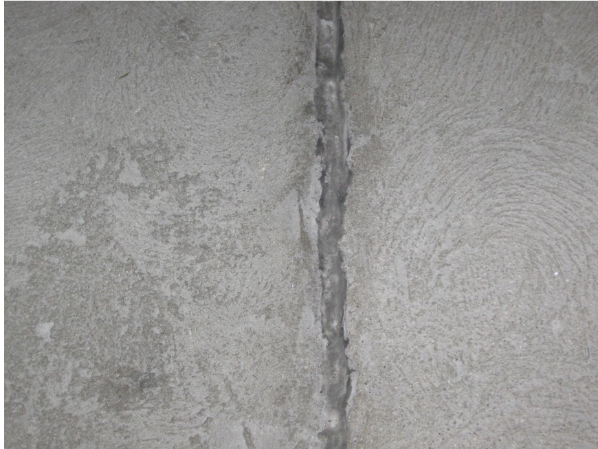
Photo 17 - Typical construction joint caulking condition
