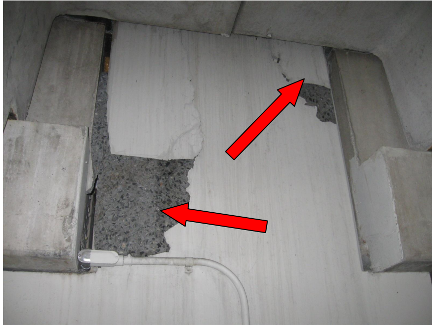
Photo 41 - Arrows denote column spalling
