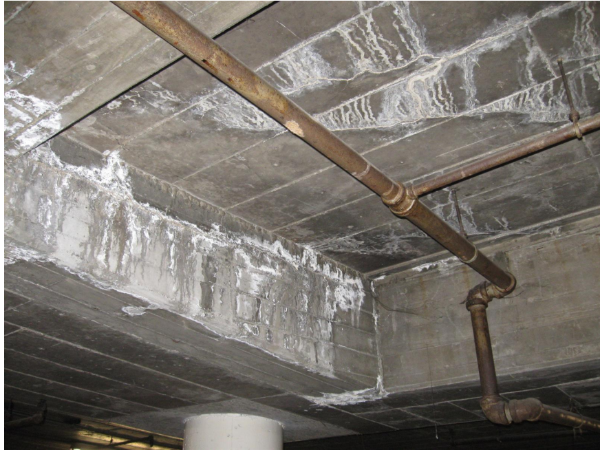
Photo 32 - Water leakage beneath entrance/exit ramps
