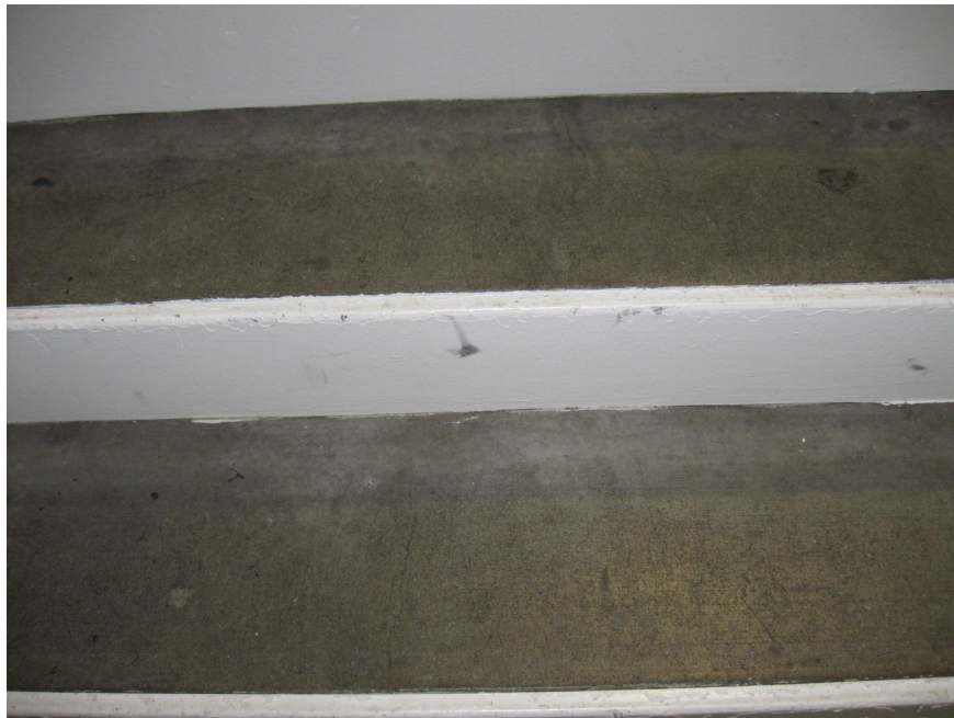
Photo 18 - Typical condition of stairwell cast-in-place treads; note random cracking
