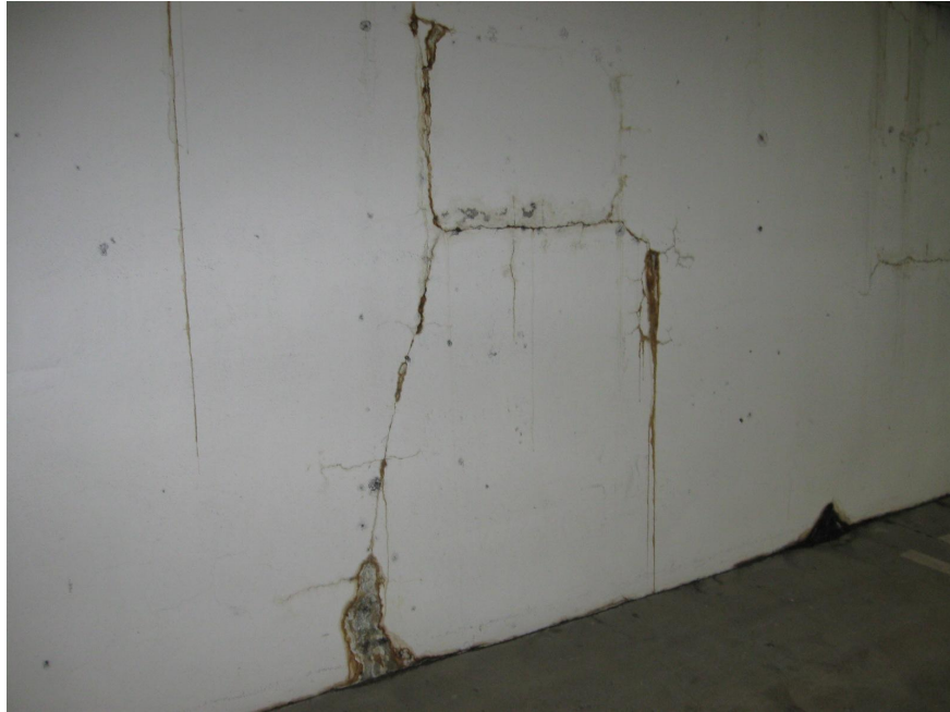
Photo 43 - Typical leaking foundation wall cracks
