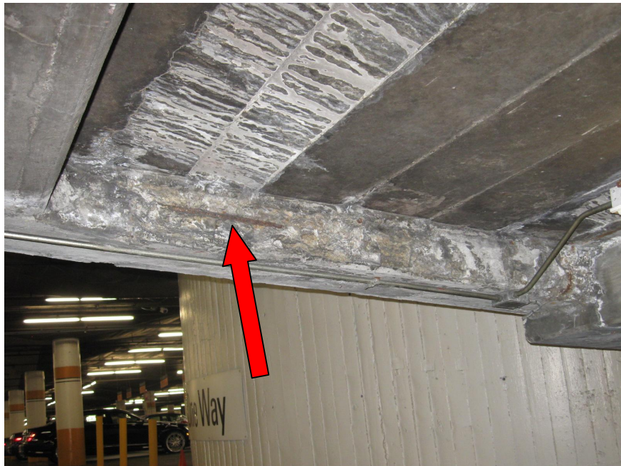
Photo 25 - Water leakage beneath entrance/exit ramps; arrow denotes beam spalling
