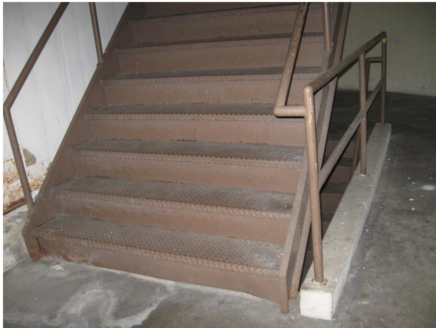
Photo 33 - Typical condition of stairs; note minor corrosion and steepness of stairs
