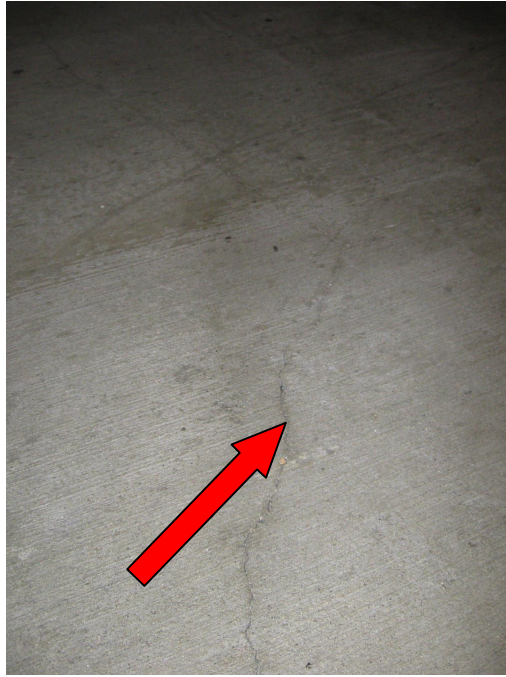
Photo 130 – Extensive slab cracking
