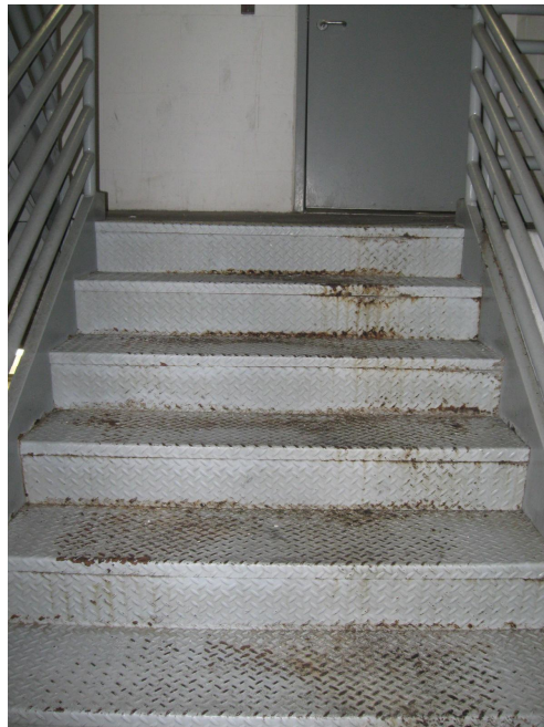
Photo 46 - Stairwell steel component corrosion
