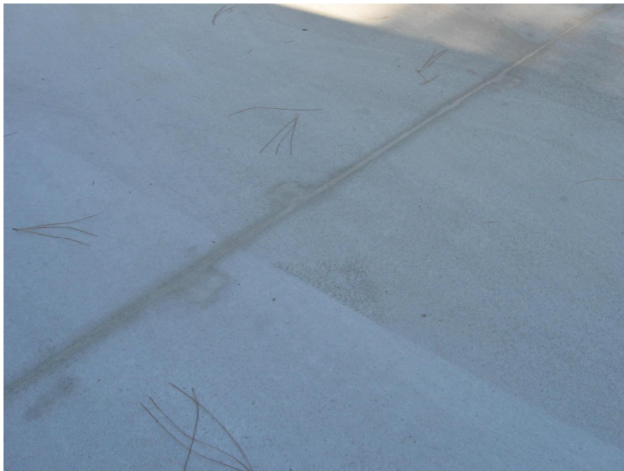
Photo 87 – Joint in concrete topping below membrane
