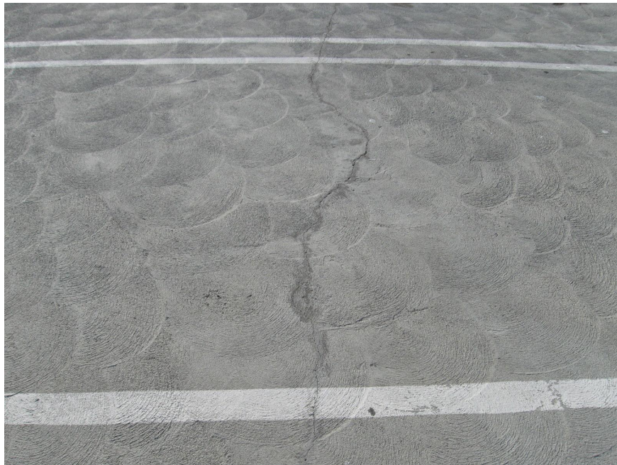
Photo 12 - Typical slab cracking on roof level
