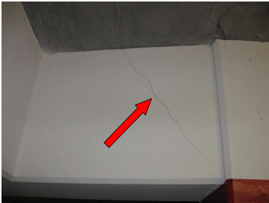
Photo 147 – Beam cracking
