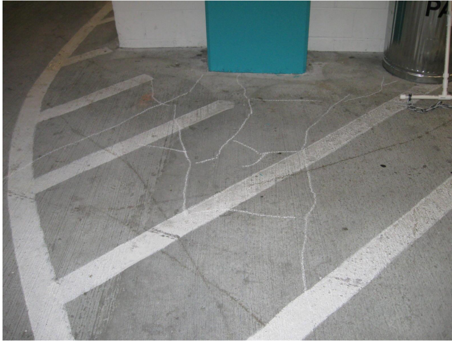
Photo 142 – Slab cracking is highlighted in chalk
