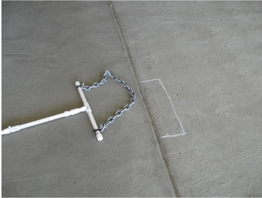
Photos 60 and 61 – Delaminated areas marked in field
