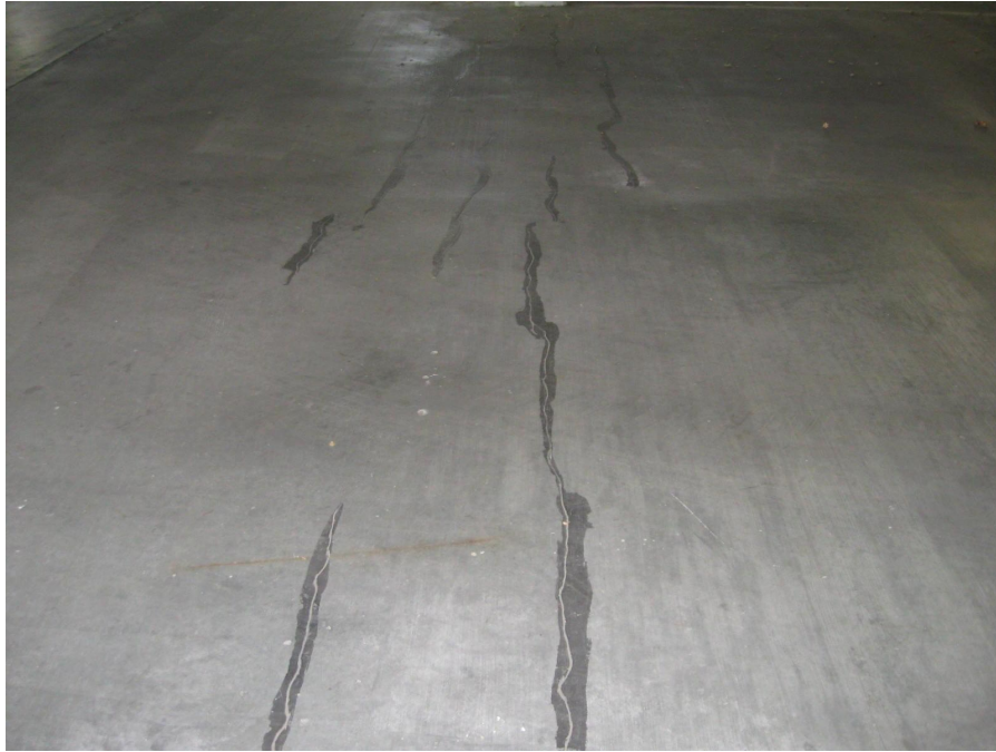
Photos 104 and 105 – Floor cracking
