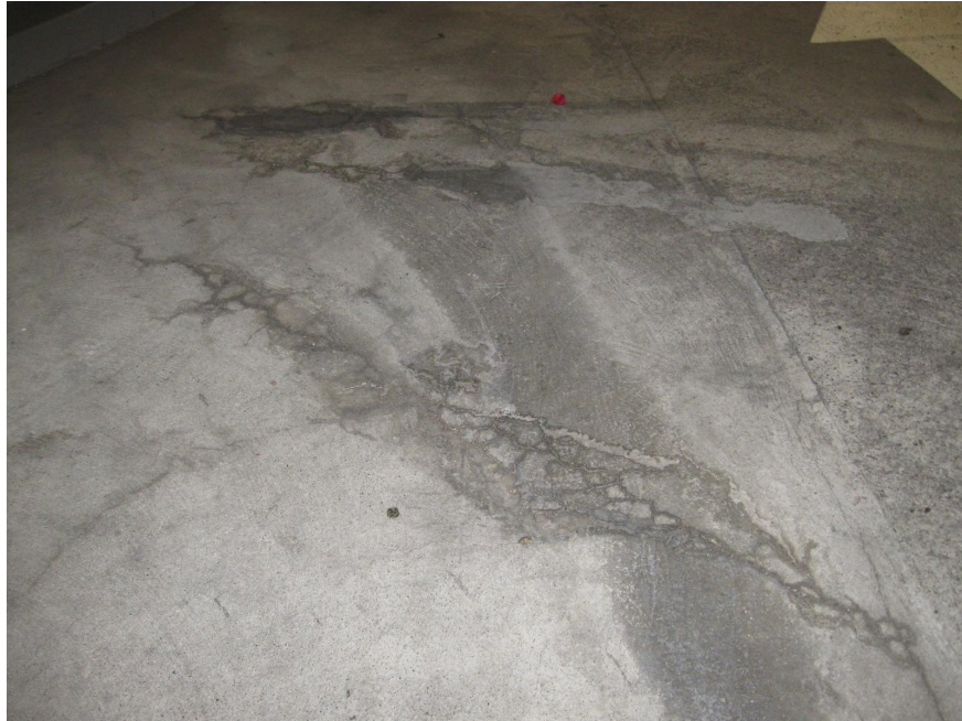
Photo 22 - Typical slab spalling/delamination
