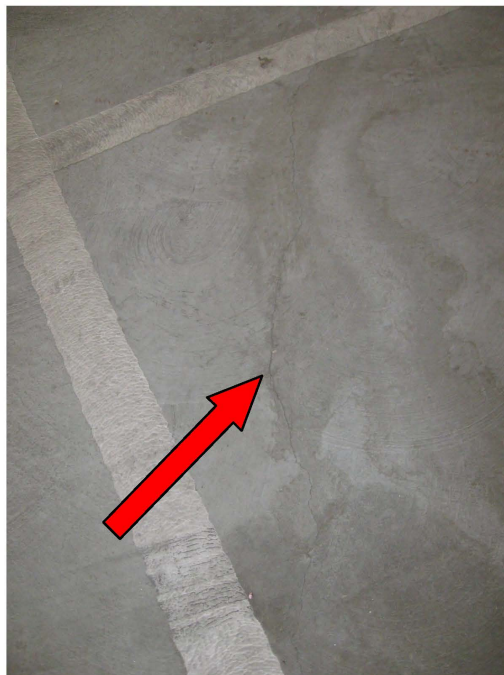
Photo 63 – Slab cracking
