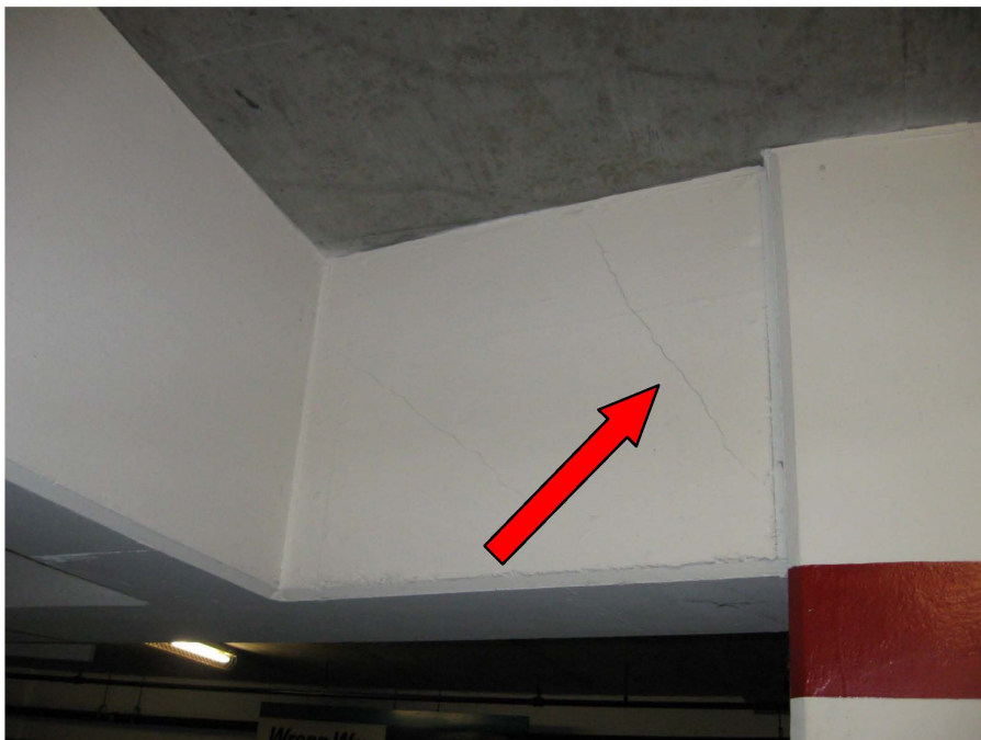
Photo 139 – Diagonal beam cracking
