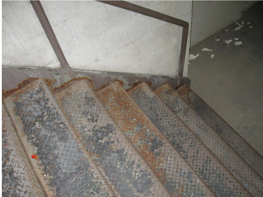
Photo 34 - Corrosion of stairwell steel components
