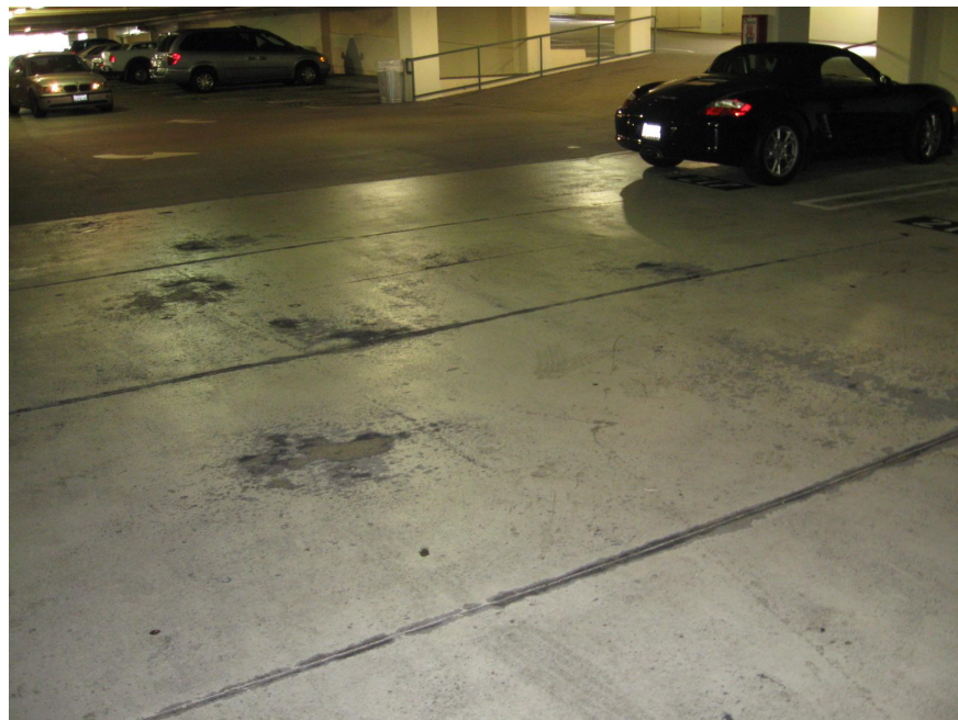
Photo 6 - Typical wear and tear of waterproofing membrane on Level 2 over retail space
