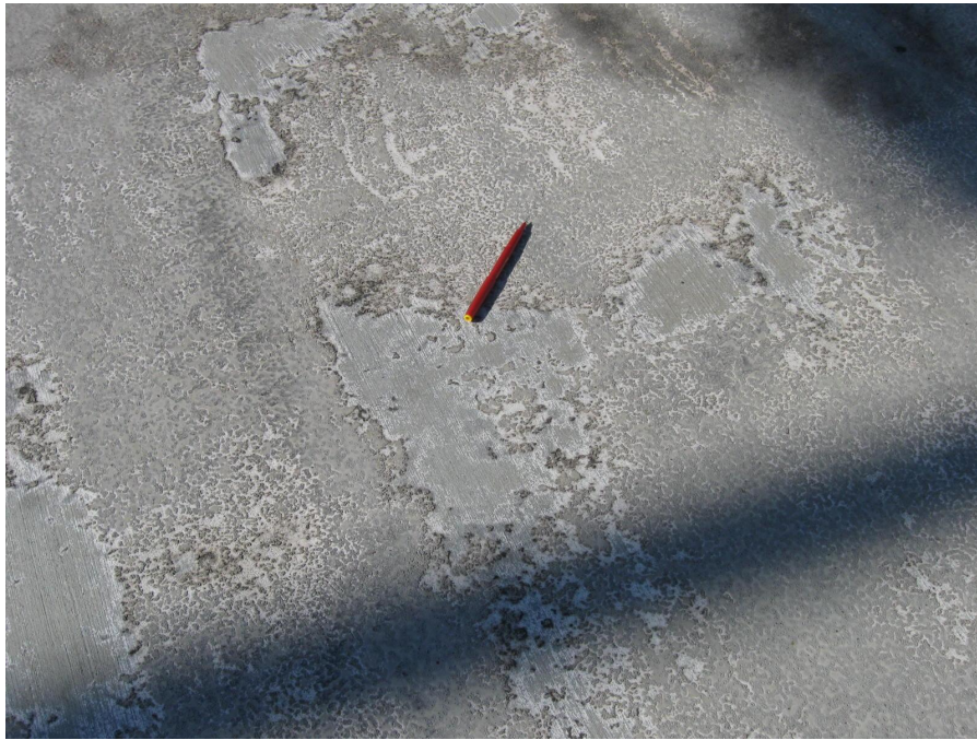
Photo 207 – Worn membrane on roof
