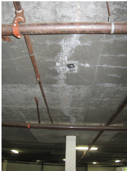
Photos 113 and 114 – Leaking slab cracks
