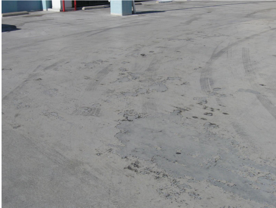
Photo 206 – Worn membrane on roof
