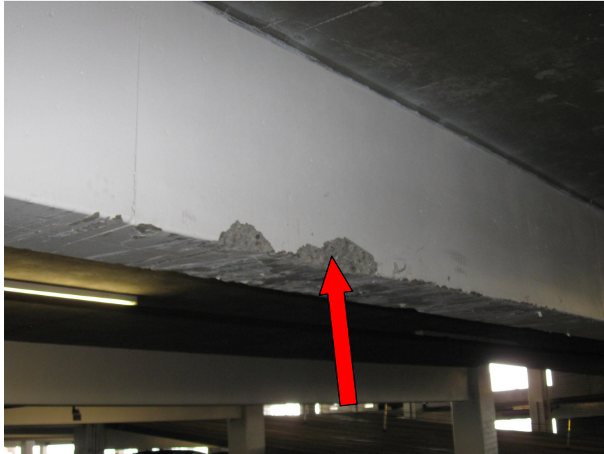
Photo 19 - Arrow denotes beam spalling at locations of apparent damage caused by oversized vehicles
