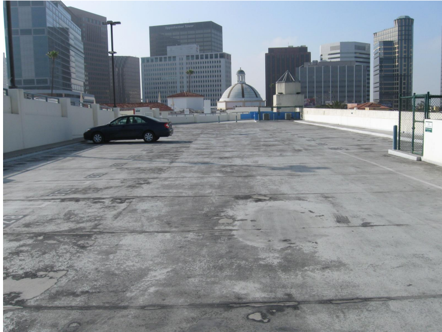
Photo 7 - Typical poor condition of roof level waterproofing membrane
