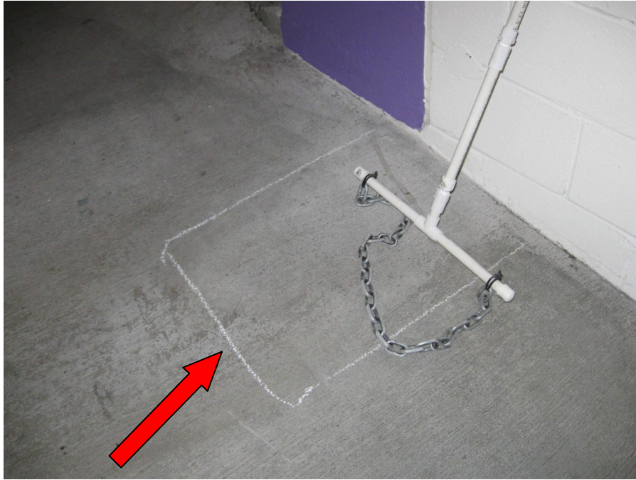
Photo 136 – Delaminated area marked
