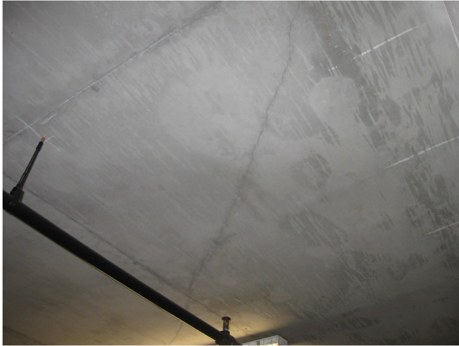
Photo 146 – Thru-slab cracking
