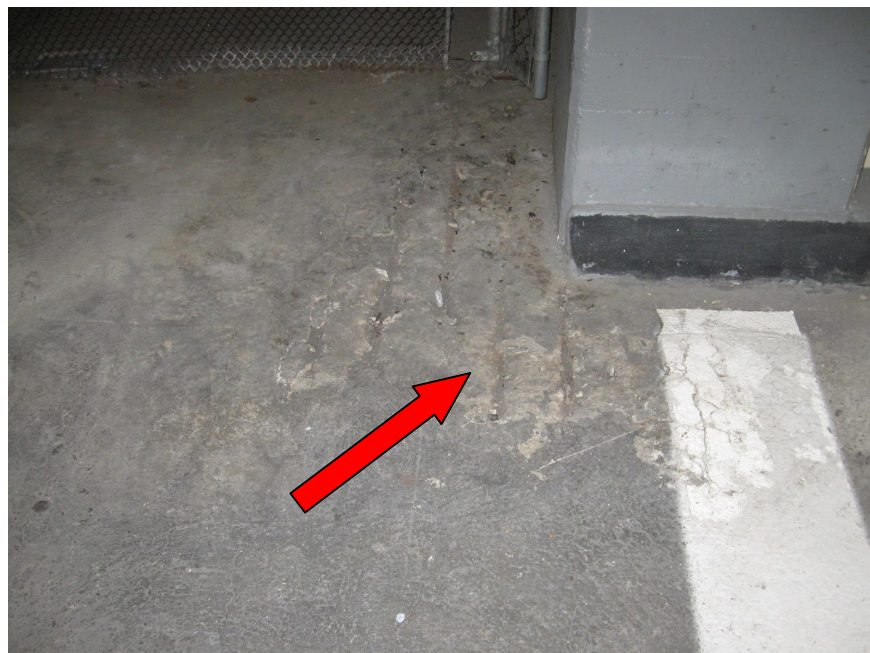
Photo 2 - Arrow denotes slab spalling/delamination
