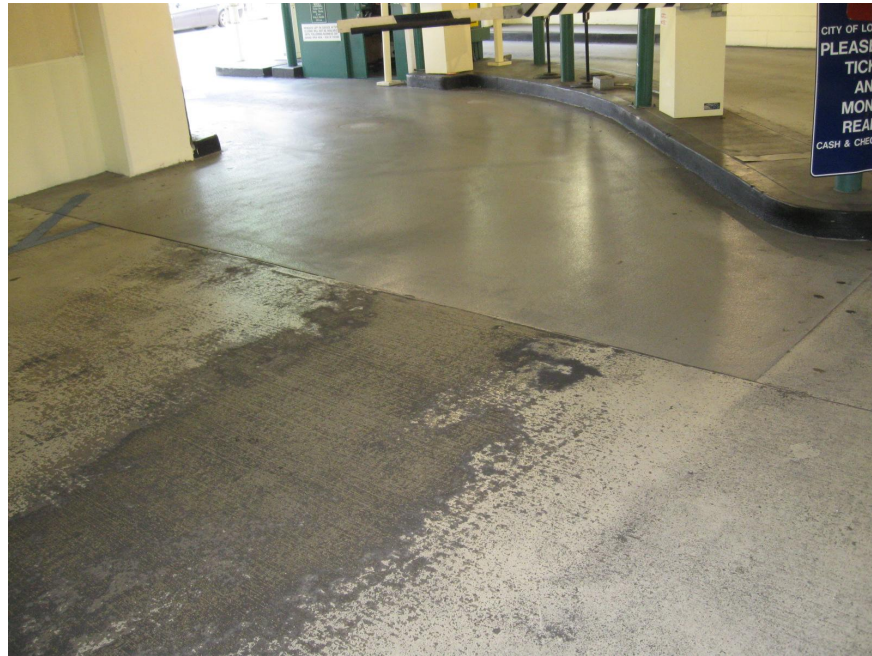
Photo 5 - Typical wear and tear of waterproofing membrane at entrance and exit lanes
