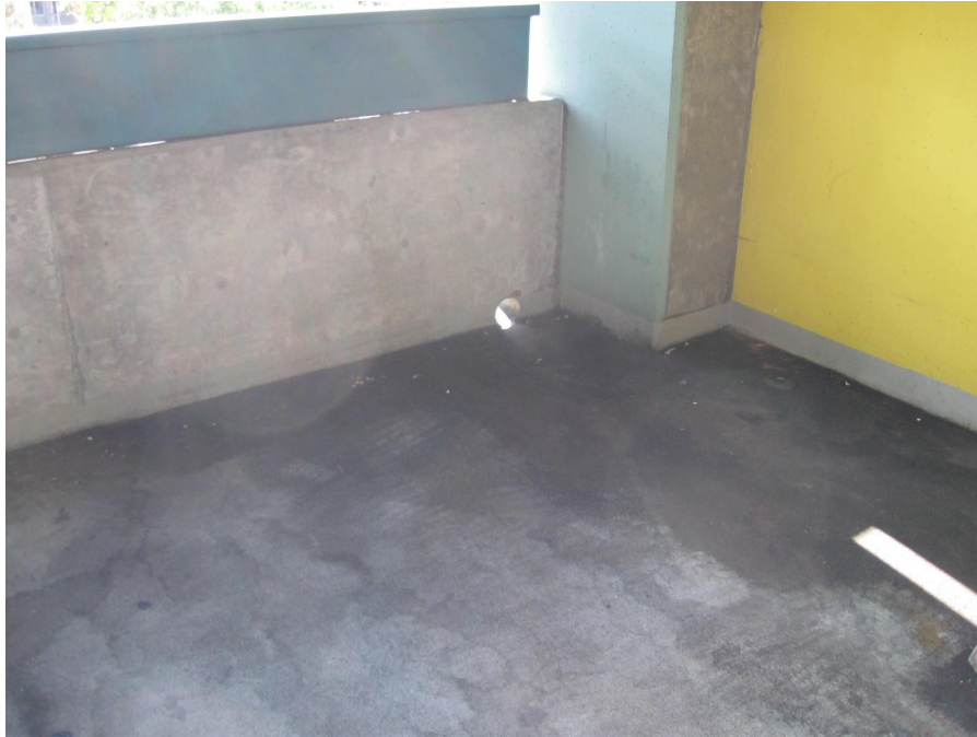
Photo 202 through 204 – Typical water ponding areas
