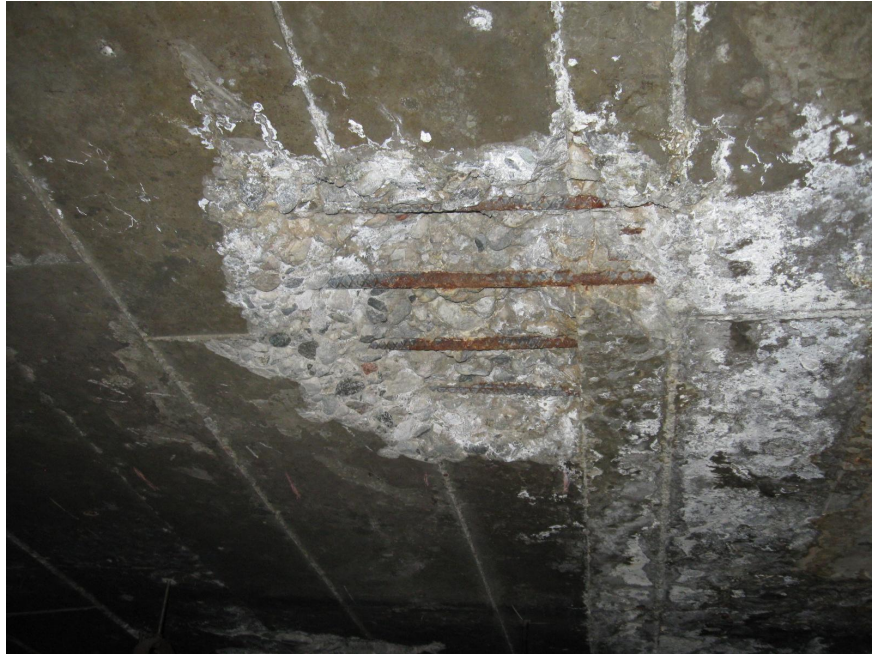
Photo 24 - Soffit spalling along construction joint
