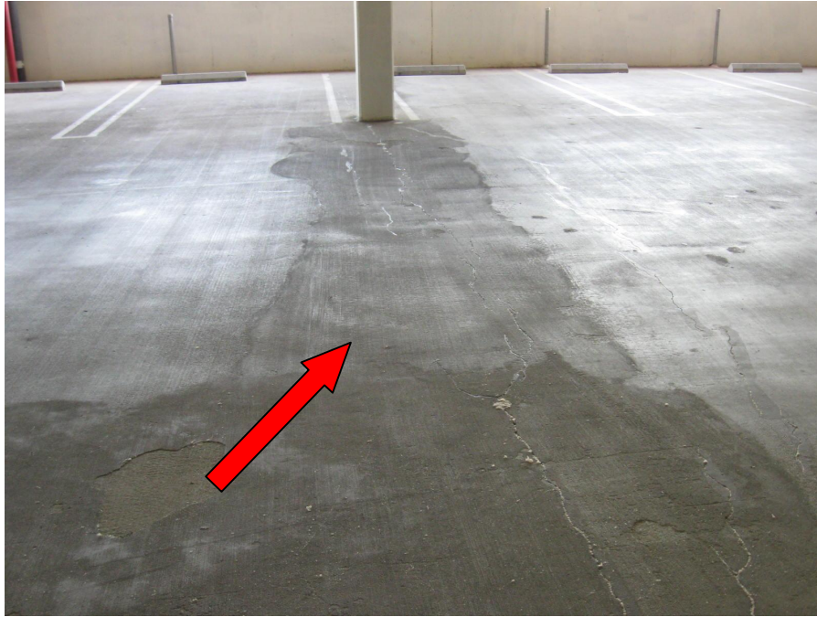
Photos 106 through 108 – thin overlay material
