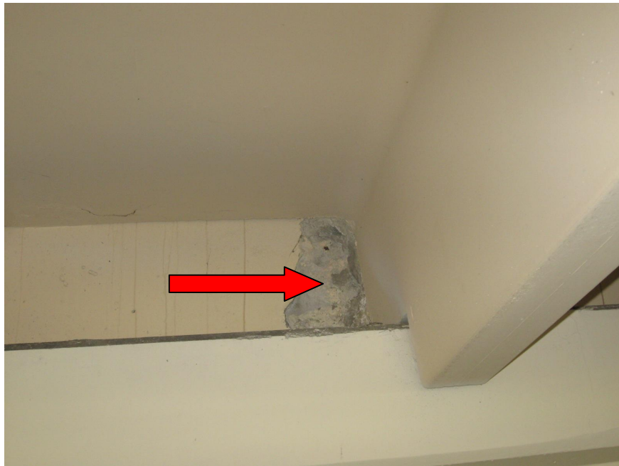
Photo 4 - Arrow denotes typical beam spall
