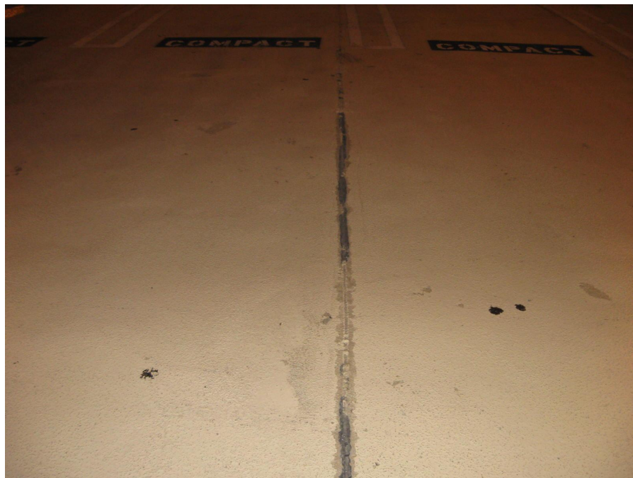
Photo 170 through 172 – Poor condition of membrane over tee joint
