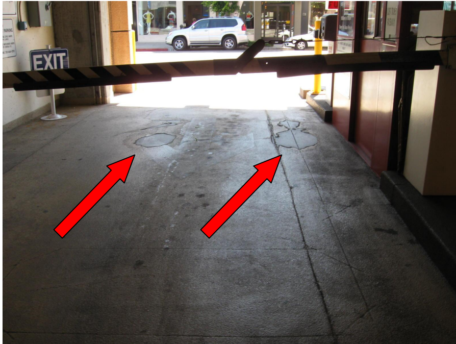
Photo 173 – Worn membrane at entrance
