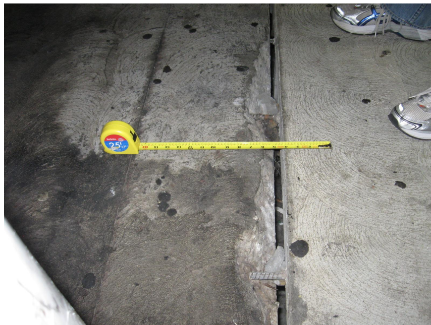
Photo 36 - Cracking along column line 5
