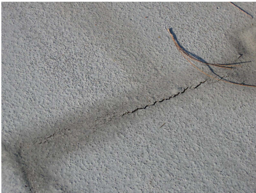
Photo 83 – Typical cracking at joints in upper level
