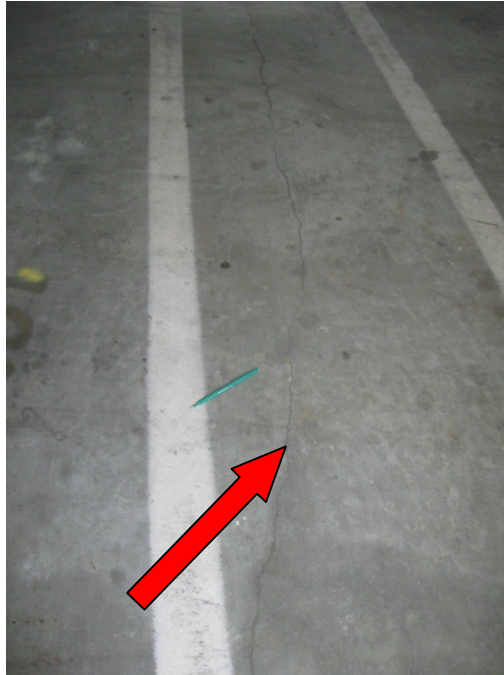
Photo 110 – Slab cracking
