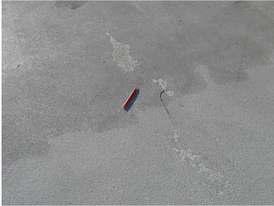
Photo 86 – Worn membrane
