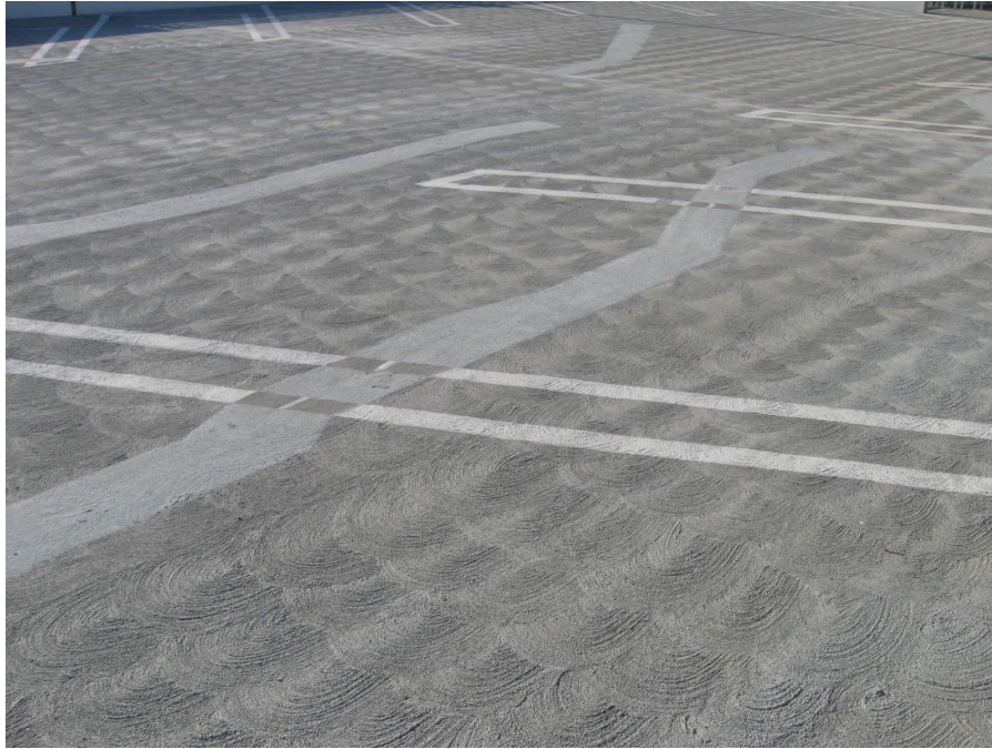
Photo 56 – Level 4 cracks previously ‘filled’
