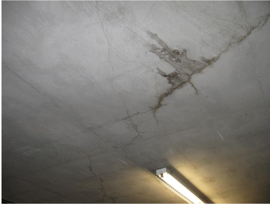
Photo 148 – Thru slab cracking
