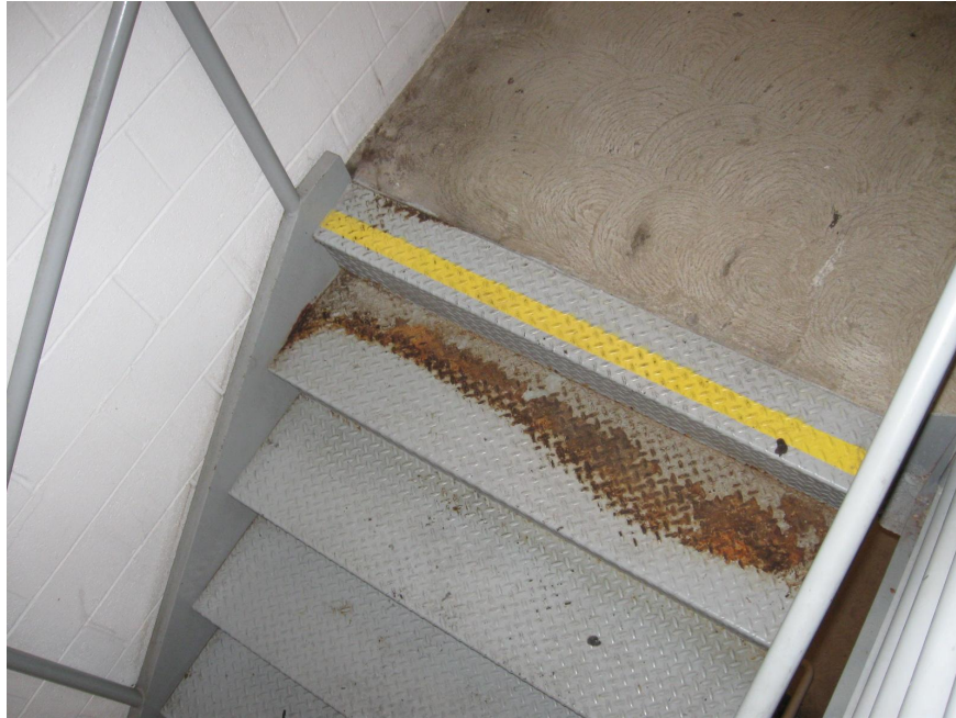
Photo 47 - Stairwell steel component corrosion
