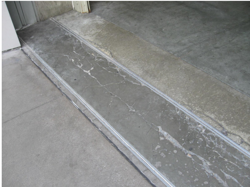
Photo 14 - Spalling at interface between garage and plaza on Level 2
