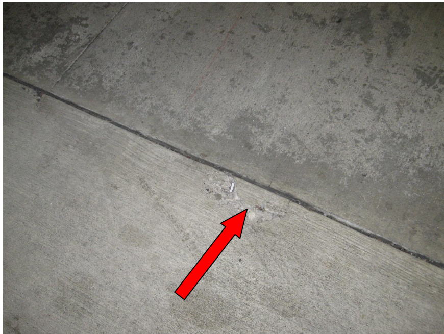
Photo 2 - Arrow denotes typical slab spall in cast-in-place concrete slab infill area
