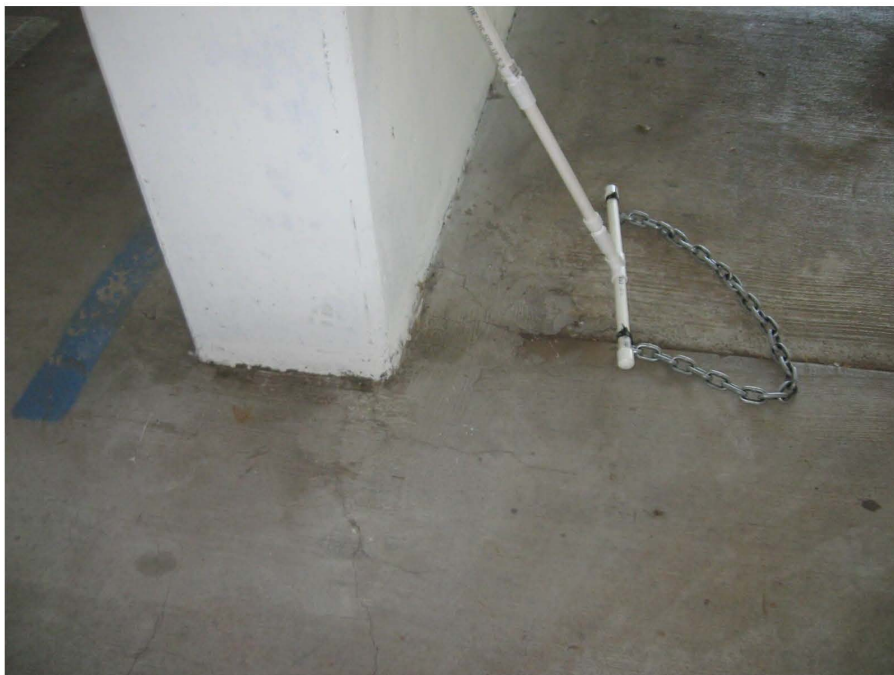
Photo 109 – Delaminated area adjacent to shear wall
