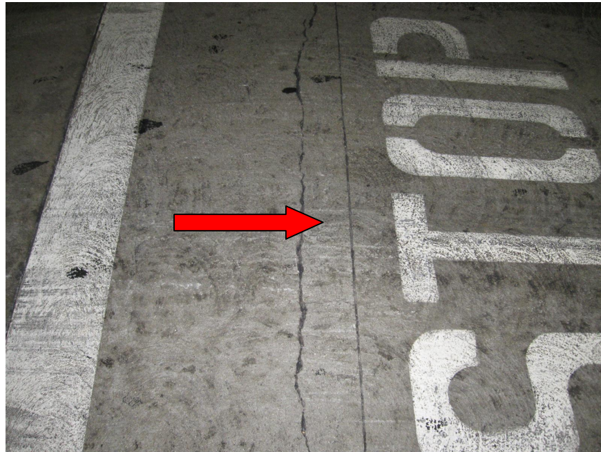
Photo 39 - Arrow denotes typical slab delamination
