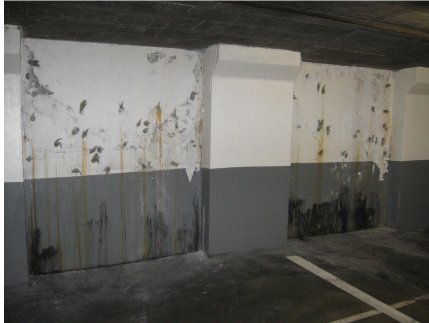
Photo 26 - Typical leaking foundation wall cracking
