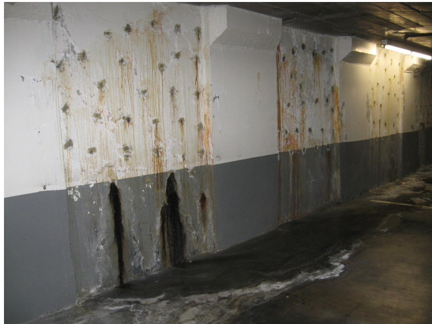
Photo 27 - Typical leaking foundation wall cracking; note previous repairs in ' Poor ' condition
