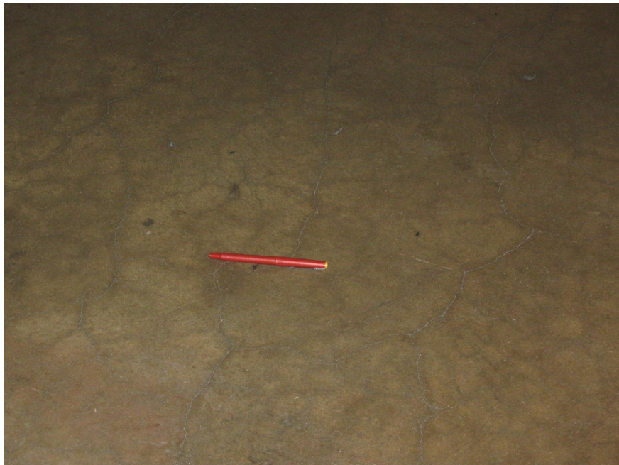
Photo 23 - Typical slab cracking
