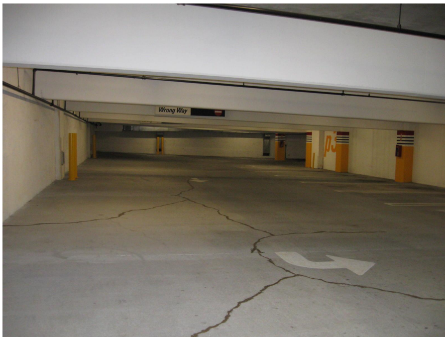
Photo 145 – Note dark, 'filled' cracks
