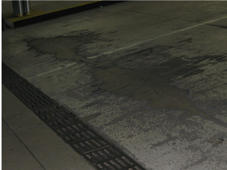
Photo 45 - Typical entrance ramp waterproofing membrane condition
