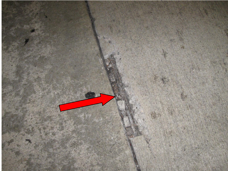
Photo 1 - Arrow denotes typical slab spall in cast-in-place concrete slab infill area
