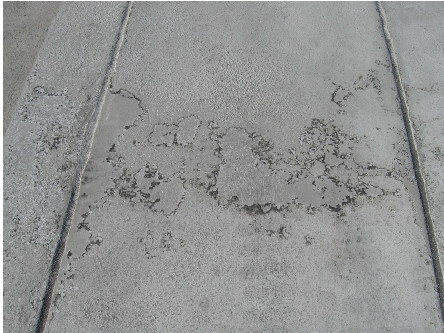
Photo 15 - Typical condition of roof level pour strip waterproofing membrane
