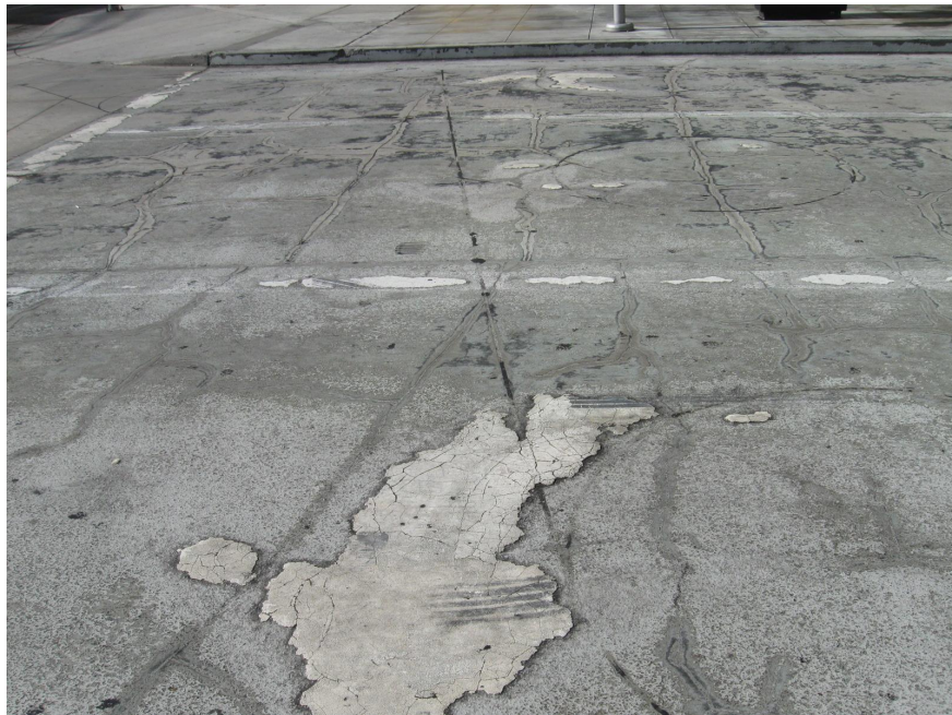
Photo 44 - Typical entrance ramp waterproofing membrane condition
