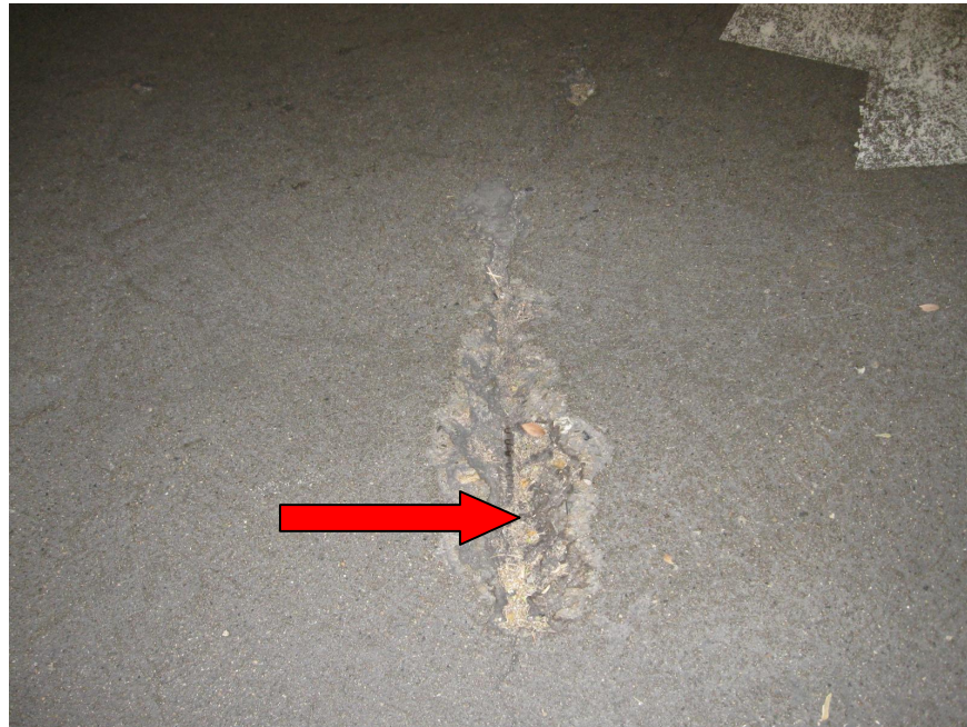
Photo 20 - Arrow denotes typical slab spalling
