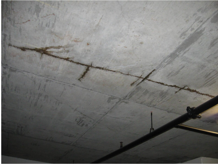
Photos 140 and 141 – Leaking cracks thru slab
