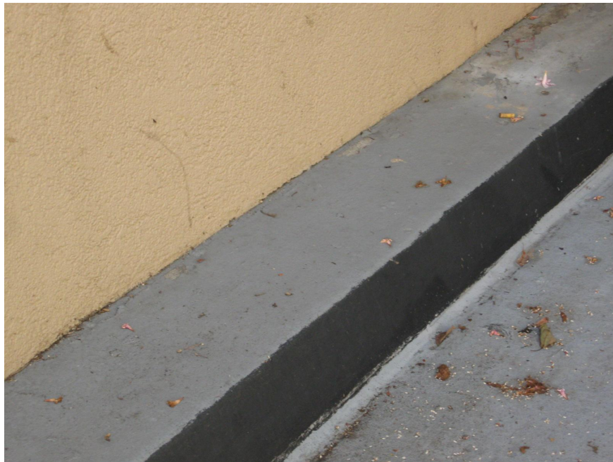
Photo 31 - Lack of flashing of waterproofing membrane at vertical terminations
