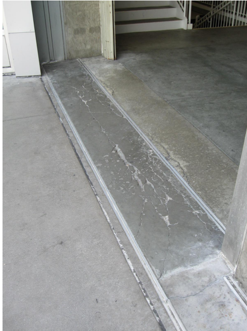
Photo 13 - Spalling at interface between garage and plaza on Level 2
