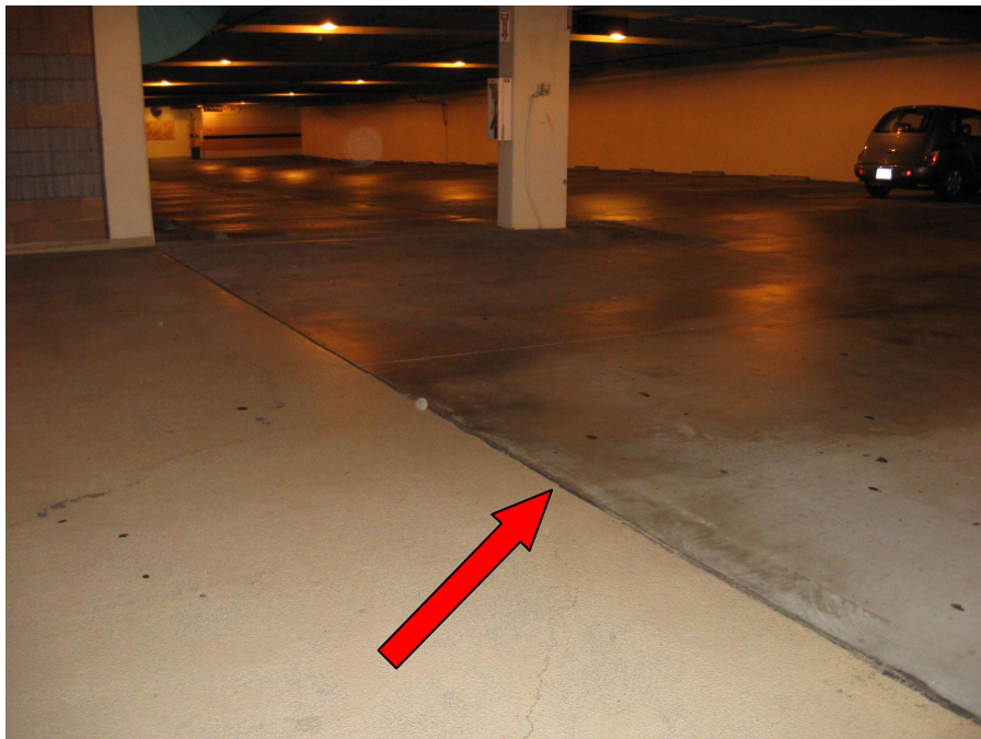
Photo 160 – Termination of waterproofing membrane system
