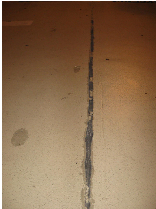
Photo 174 through 178 - Poor condition of membrane over tee joint
