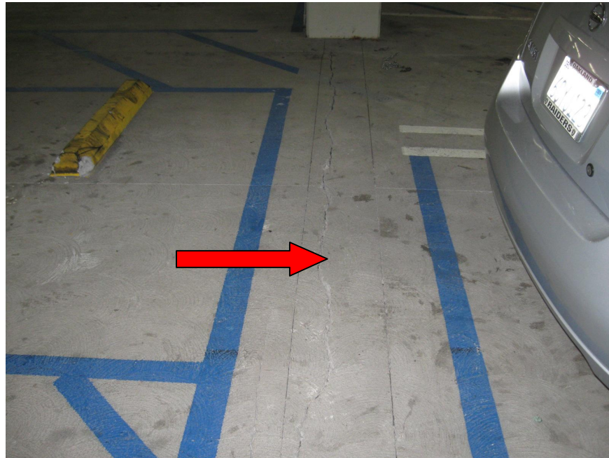
Photo 35 - Arrow denotes typical cracking along column line 5
