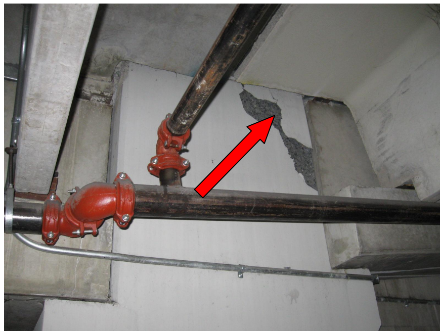
Photo 40 - Arrow denotes column spalling
