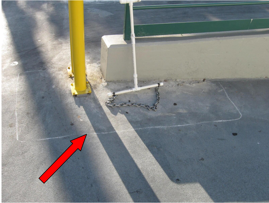
Photo 126 – Delaminated area is marked
