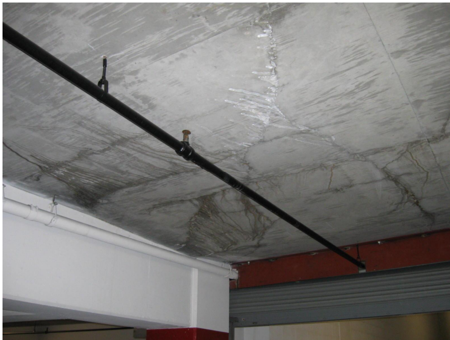
Photo 149 – Thru slab cracking
