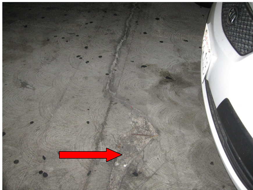
Photo 38 - Cracking along column line 5; arrow denotes spalling
