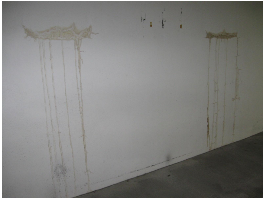
Photo 42 - Typical leaking foundation wall cracks
