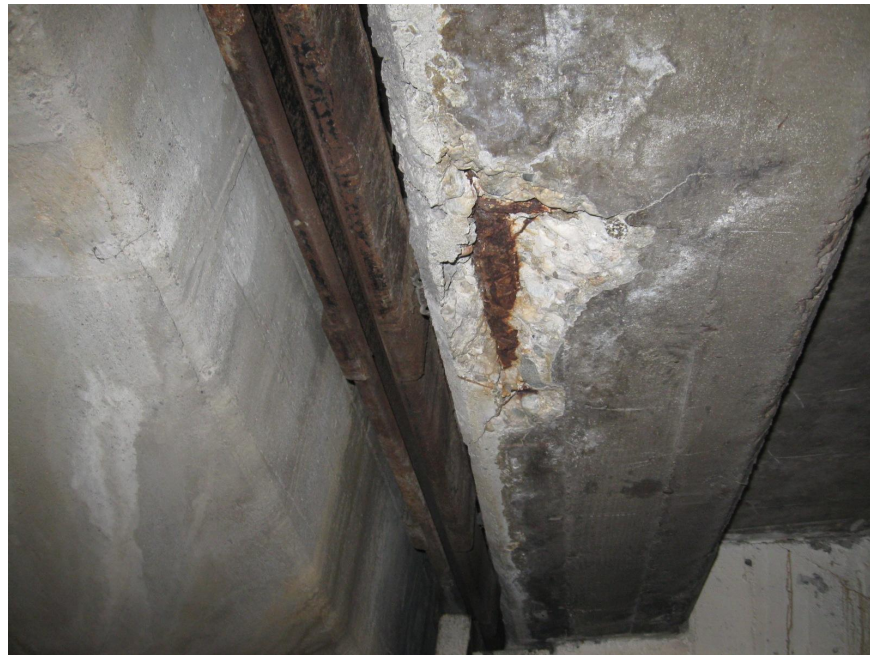
Photo 29 - Signs of leakage and beam spalling directly beneath expansion joint assemblies
