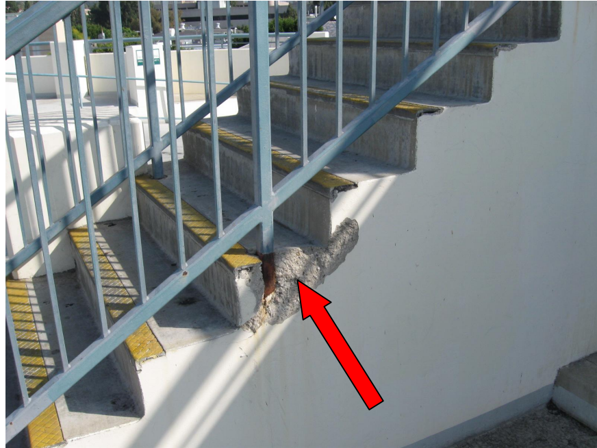
Photo 9 - Arrow denotes stair tread and riser spalling
