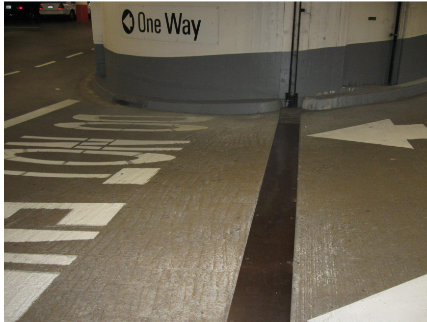
Photo 28 - Typical steel expansion joint assembly
