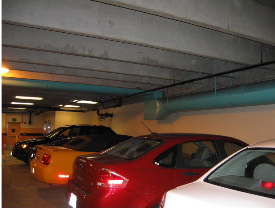
Photos 161 through 164 – Double tee component of struct. system
