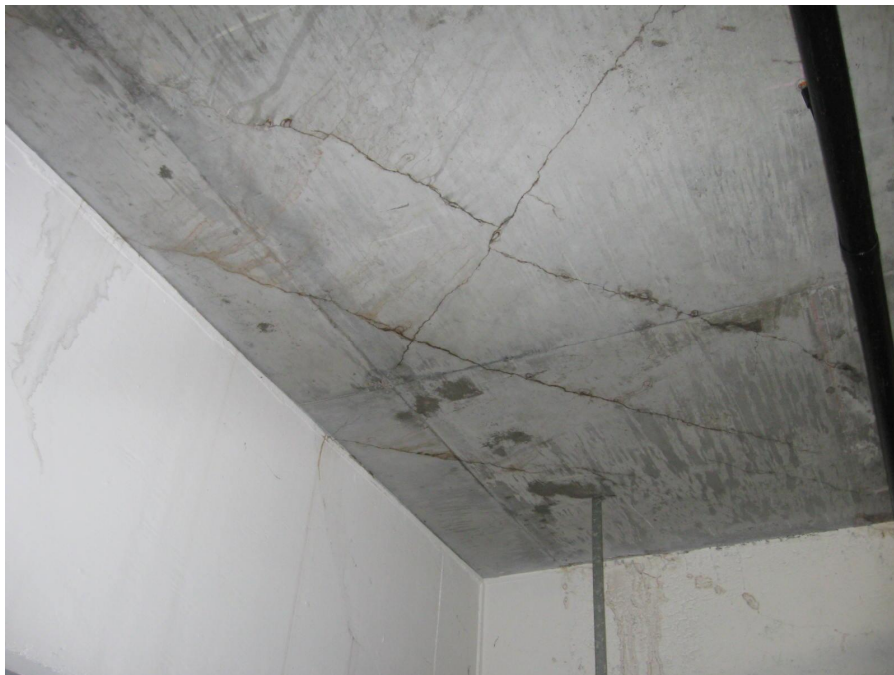
Photo 143 – Restraint cracking at corner
