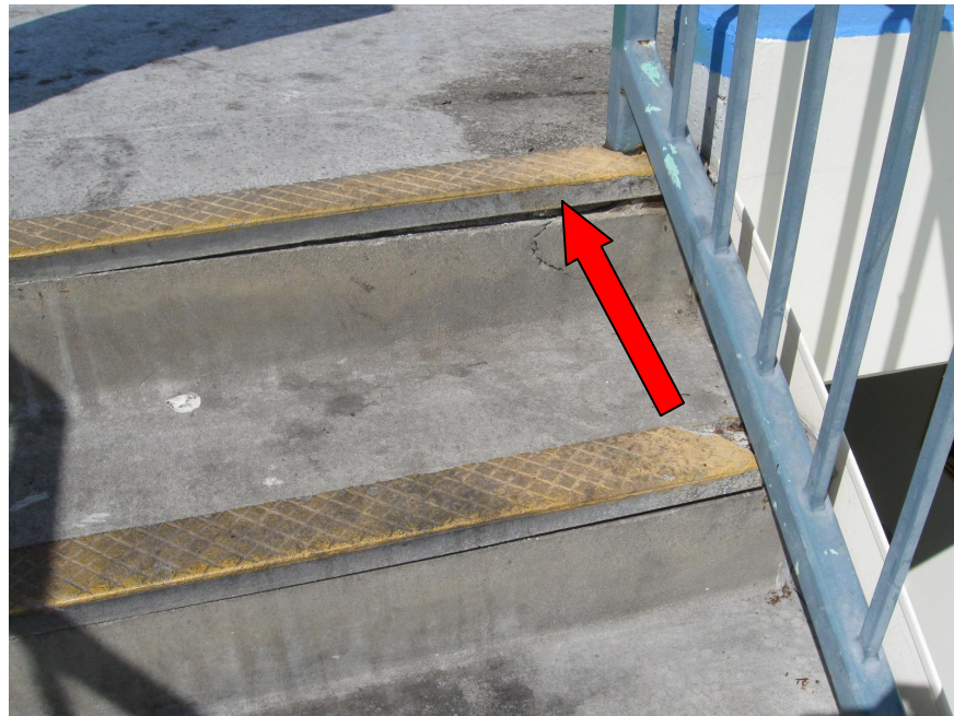
Photo 10 - Arrow denotes loosening nosing strip in stairwells
