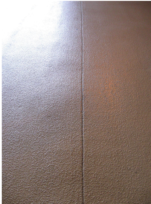
Photo 169 – Excellent condition of membrane over tee joint
