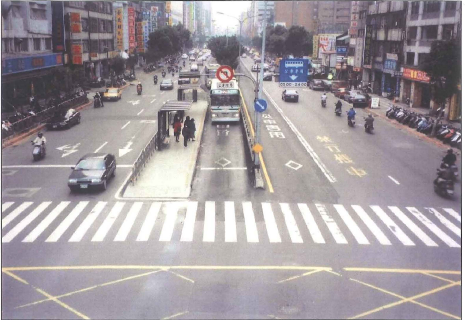
Median Busway in Taipei, Taiwan
