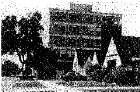
The lack of transition between commercial buildings and single-family housing shown here is no longer permitted
