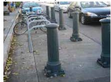
Berkeley installed architectural bollards on a concrete pad.
