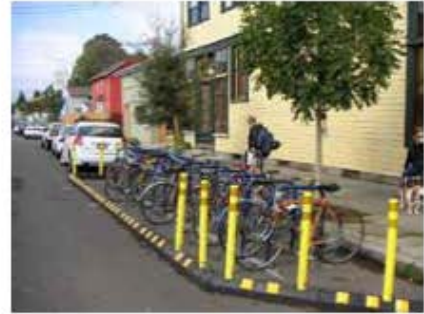
At first, Portland’s bike corrals were completely enclosed by rubber curbs with flexible bollards at either end, but this design made it difficult for cyclists to enter from the street.
