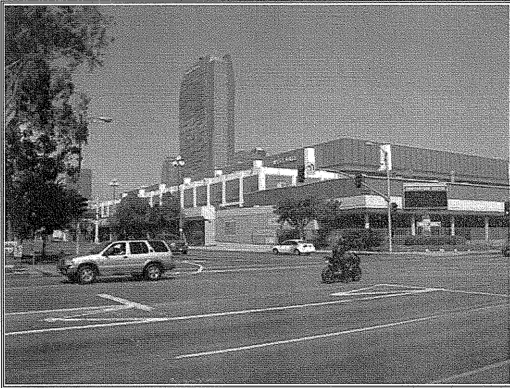
SUBJECT PROPERTY LOOKING NORTHEAST FROM PICO BOULEVARD
