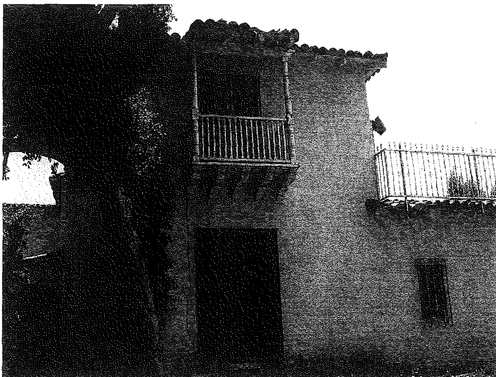
Clifford E. Clinton Residence, Western facing balcony, 5470 Los Feliz Boulevard, June 1, 2010 (Photograph by Charles J. Fisher)
