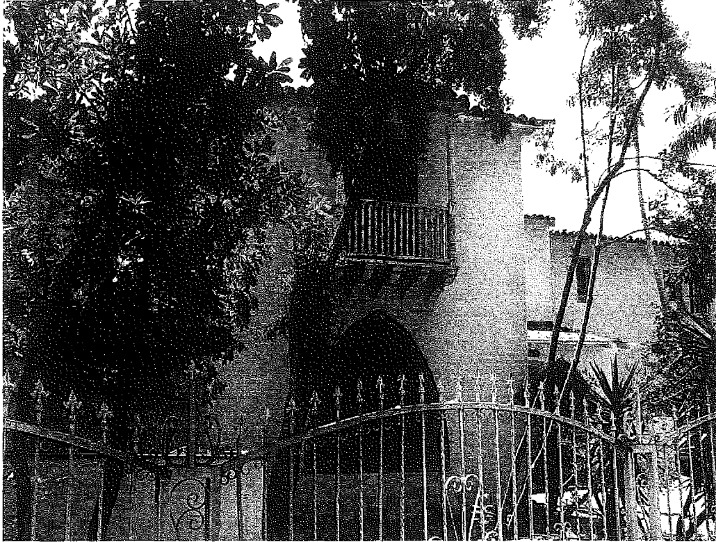
Fritz Clifford E. Clinton Residence, Los Feliz facing balcony, 5470 Los Feliz Boulevard, June 1, 2010 (Photograph by Charles J. Fisher)
