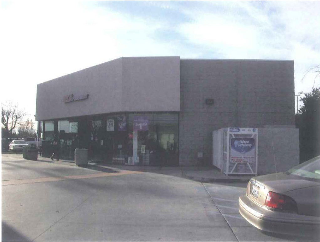
D. Looking westerly from parking lot of Site toward minimart.
