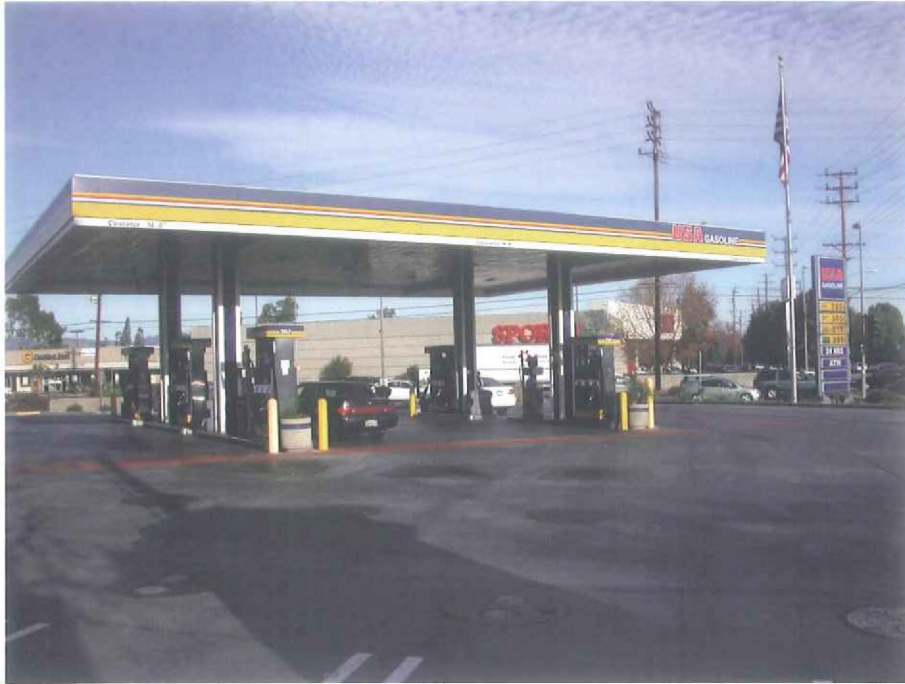
E. Looking easterly across Parthenia toward gas sales area, Sports Authority.
