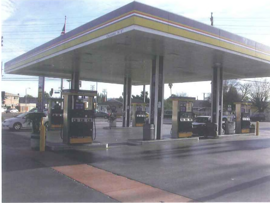
A. Canopy over gas sales area looking southerly.
