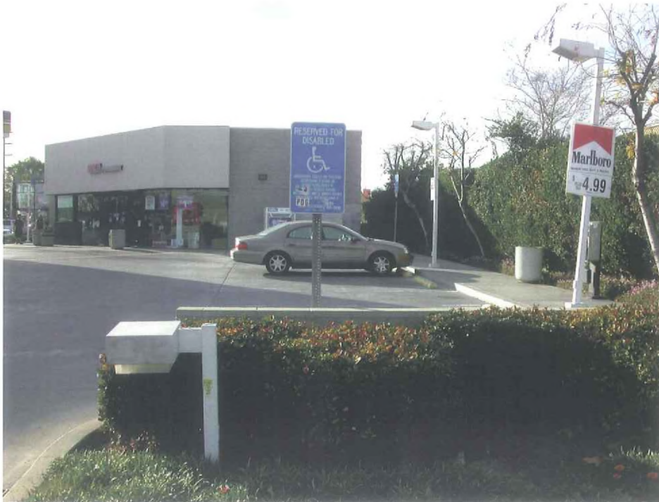
C. Looking westerly at Site from adjacent sidewalk on Tampa.
