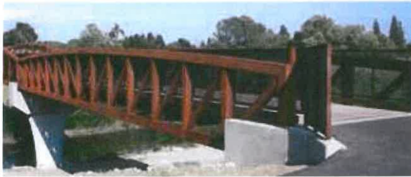
Diagram 2: Typical Steel Truss (H-Section Type) Pedestrian Bridge
