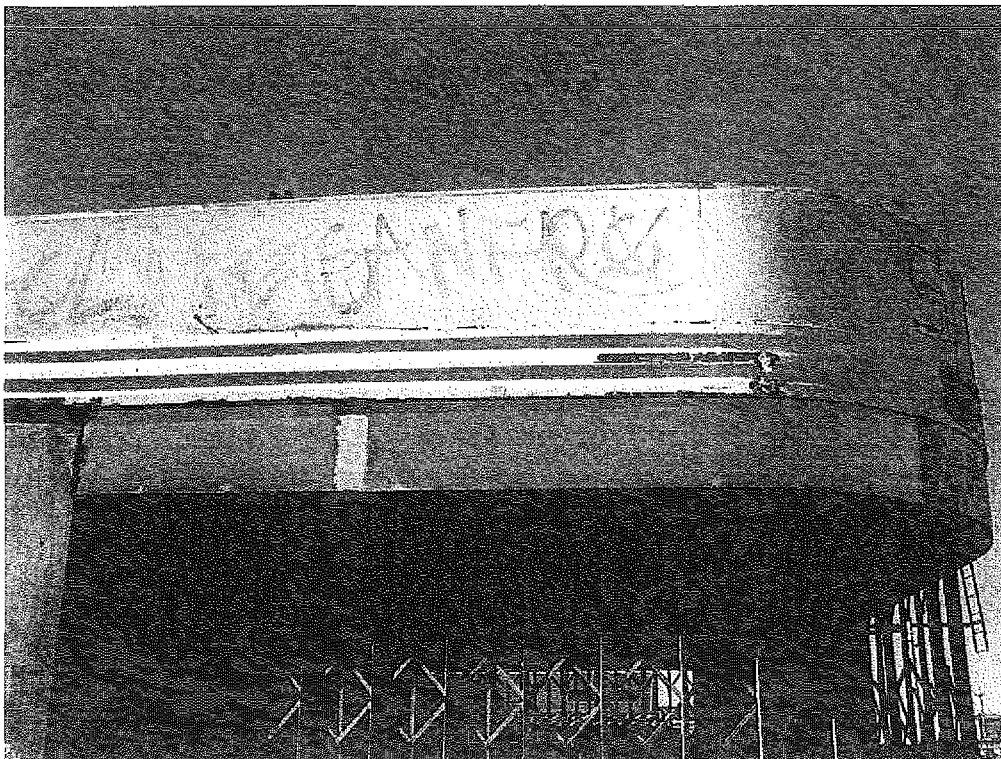
Whittier's Texaco Station, restored steel on lubrication building, 4450 Beverly Boulevard, February 9, 2011 (Photograph by Charles J. Fisher)
