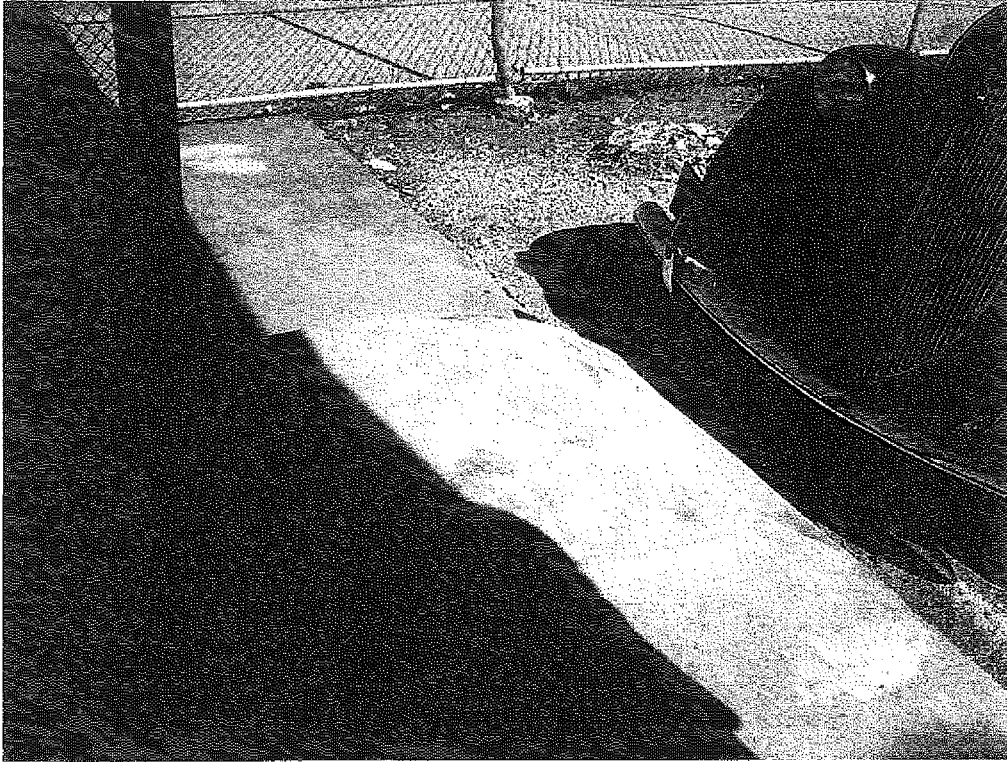
Whittier's Texaco Station, restored concrete on pump island, 4450 Beverly Boulevard, February 9, 2011 (Photograph by Charles J. Fisher)
