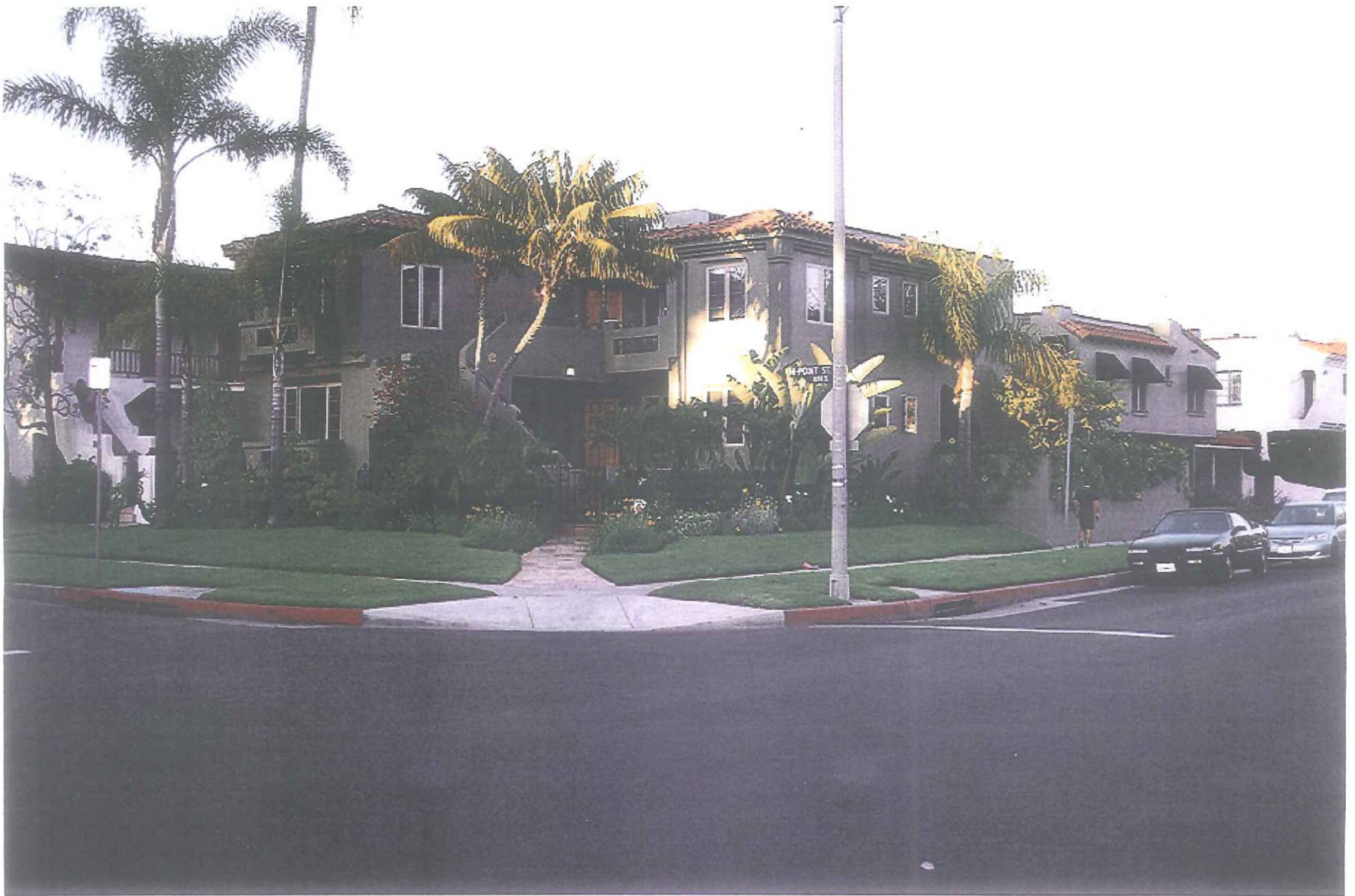
Comparable 3-unit Building at Hi Point Street and Packard Street
