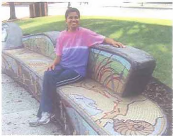
Example Mosaic Bench. Concrete planter/bench backs and concrete seat rounds will include mosaic tile in manner similar to this image. Contractor to provide surface and bed needed for mosaic in direction of project mosaic artist.
