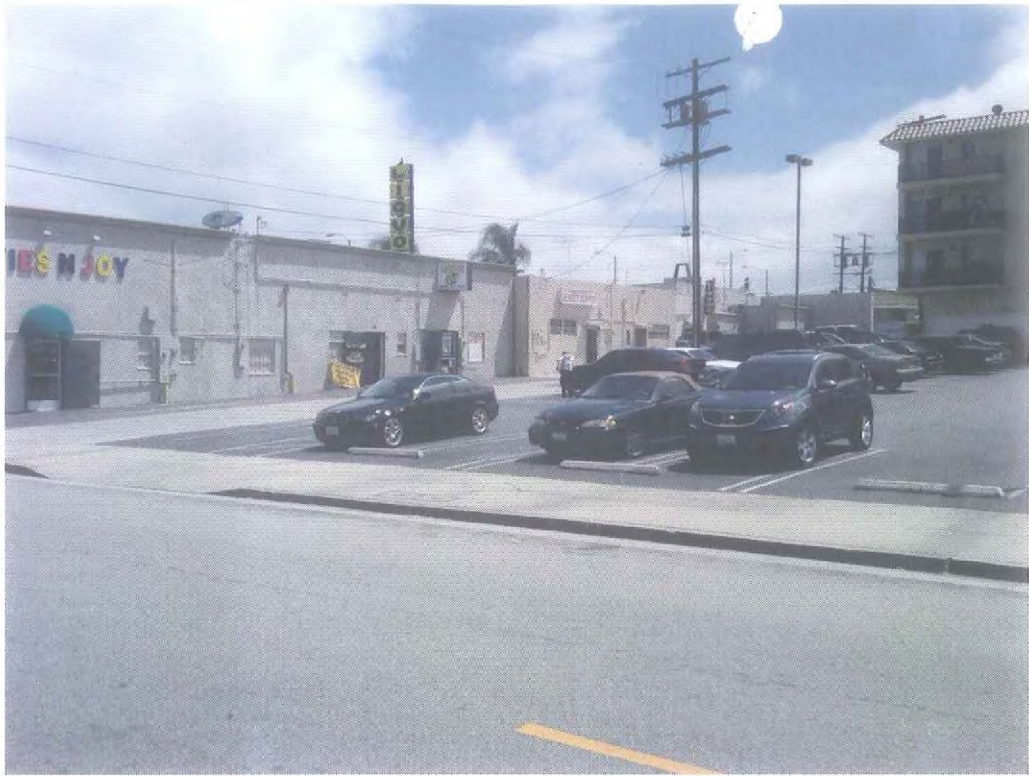
Rear of project and surface parking
