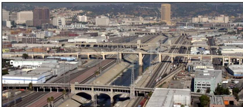
reaction called Alkali Silica Reaction (ASR), which is caused by the reactive aggregate used in the concrete. Because of this ongoing and irreversible chemical action, the 6<sup>th</sup> Street Viaduct's concrete has lost significant strength, and the structure is subject to failure under predictable seismic energy releases. The viaduct also has design deficiencies consisting of cracking and
