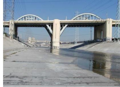
**East Approach Spans:** The east approach is similar in construction to the west approach. It has 31 spans between the east river pier and the east abutment. The span lengths and skew angles to the bents vary to allow several local streets to pass underneath the viaduct. Columns of Bent 12 are supported on pile foundations, whereas columns in all other bents are supported on spread footings.
