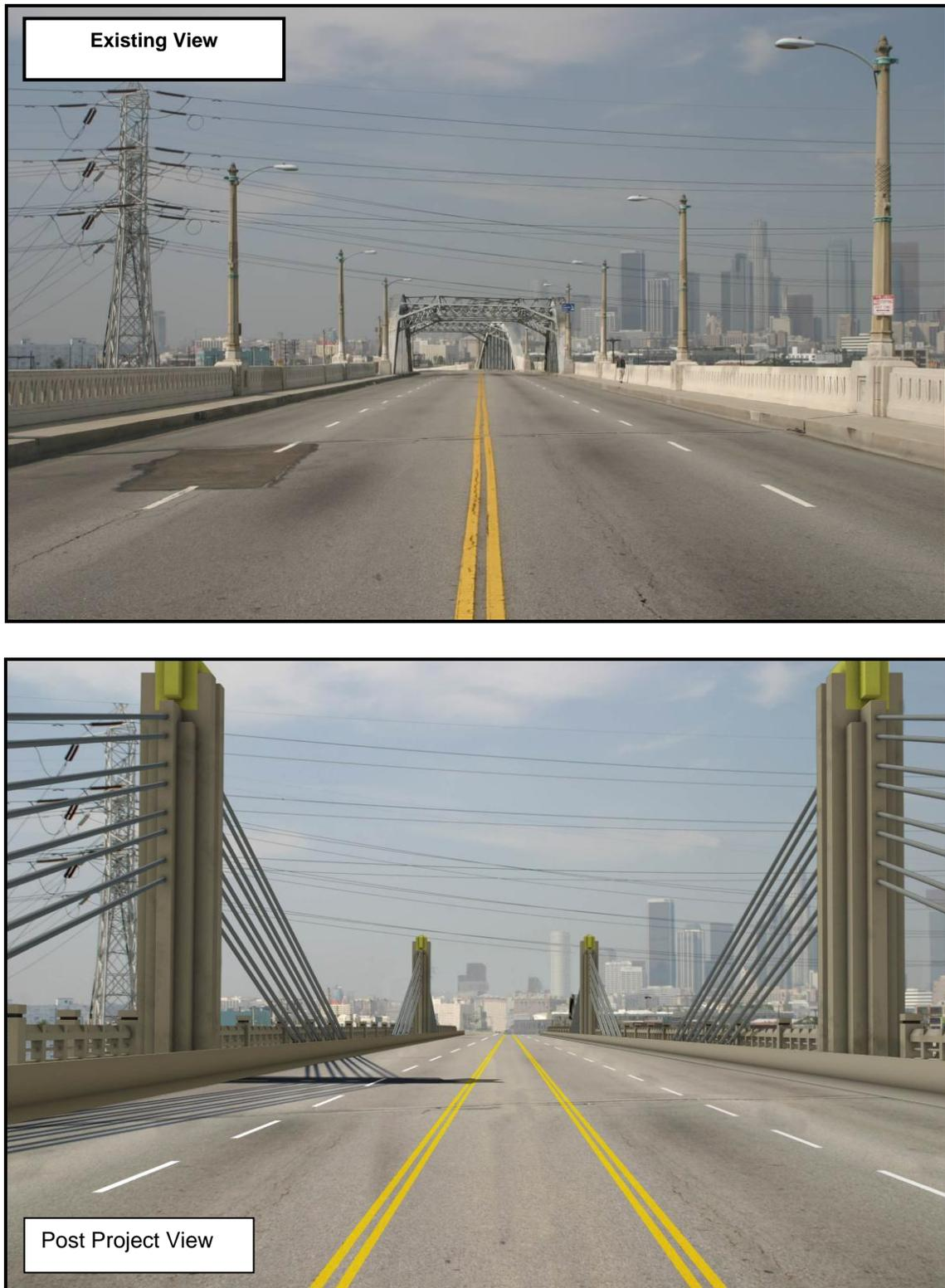
Figure 3.8-13 Viewpoint 4: Bridge Concept 4A – Extradosed with Dual Pylons
