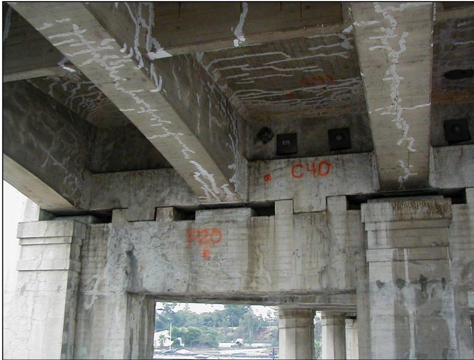
**Figure 1-6 Cracks due to ASR**
