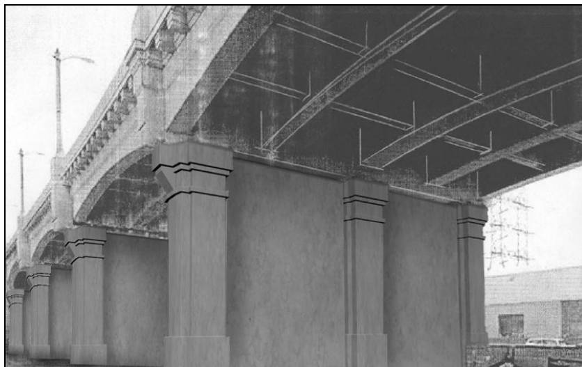
View after Retrofitting (showing a sample of in-fill wall at one column)
