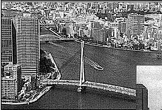
Sumida River Bridges 26 Arch Structures in 27 km
