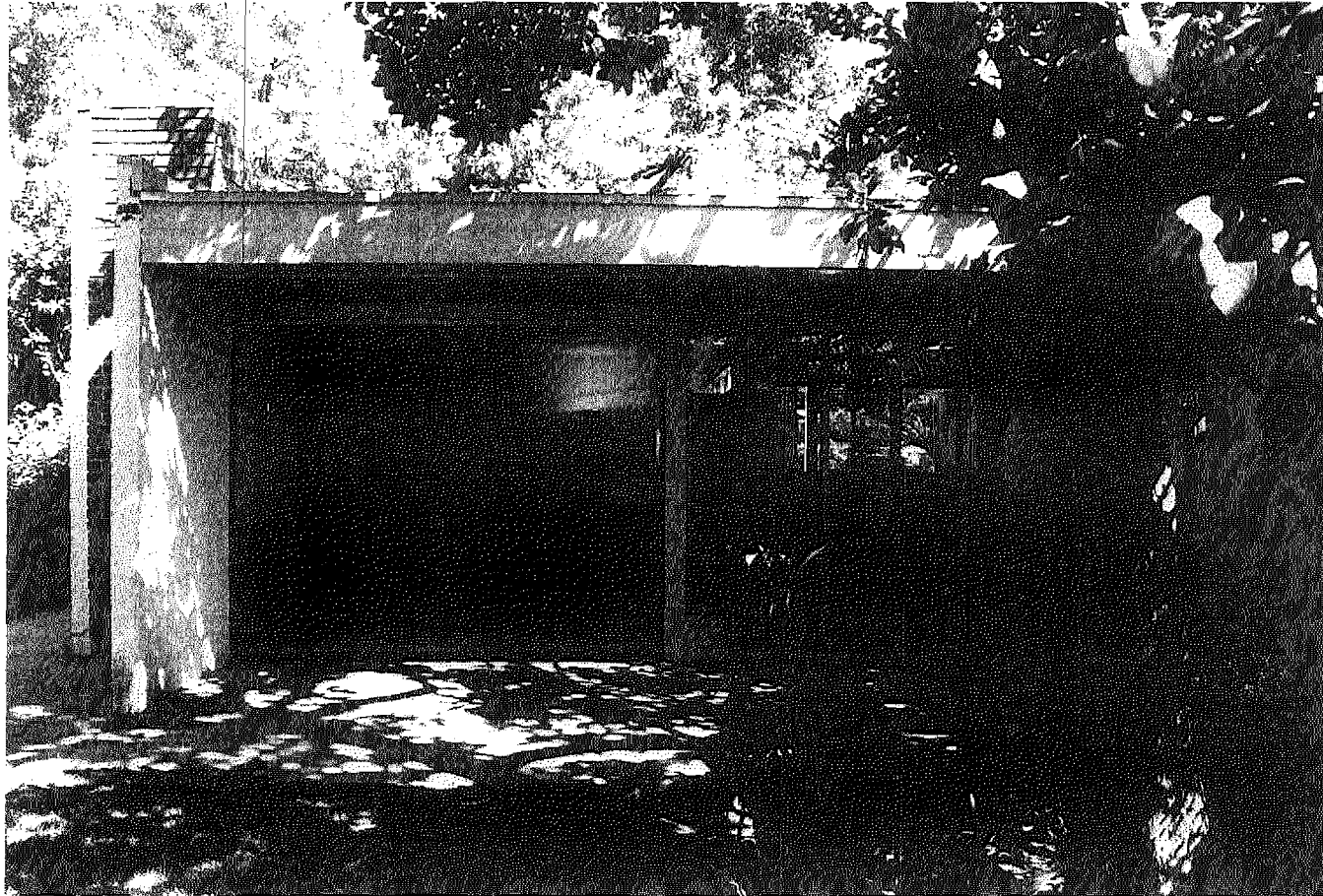
Northwest elevation, looking southeast. Photographer Laura Orozco. 20 August 2011.
