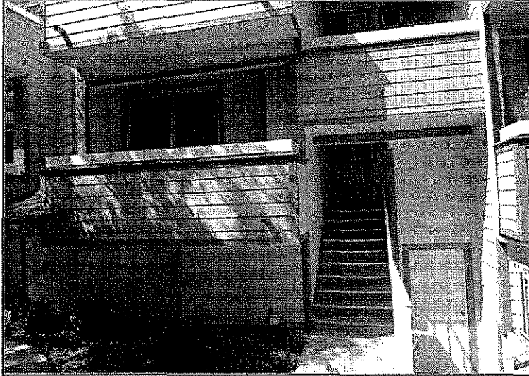
FRONT OF BUILDING @ UNIT
