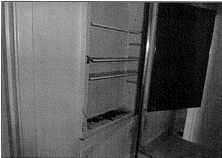
REPLACE MEDICINE CABINET
