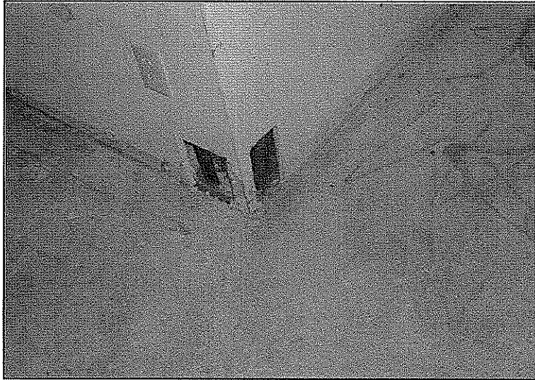
DRYWALL DAMAGE @ LIVING ROOM
