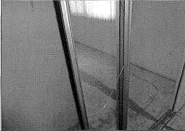
BROKEN MORRORED CLOSET DOOR @ BEDROOM
