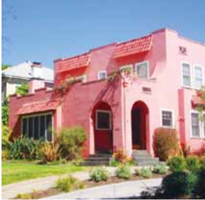
A portico creates a clear transition space between indoor and outdoor.
