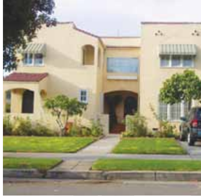
Front porches are a transition between semi-public and semi-private space.
