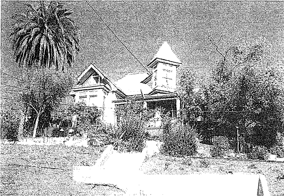
Young-Gribling Residence, 3320 Griffin Avenue, September 2, 1991 (Photograph by Charles J. Fisher)
