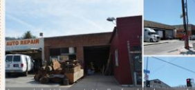
As some industrial areas start to allow for a broader range of recreational amenities will be needed, providing pedestrian-friendly sidewalks, on-site open space and on-street parking.
