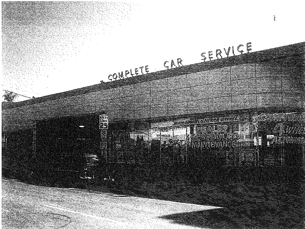
Firestone Tire Building, 8 th Street facade, 800 S. La Brea Avenue, October 29, 2011 (Photograph by Charles J. Fisher)
