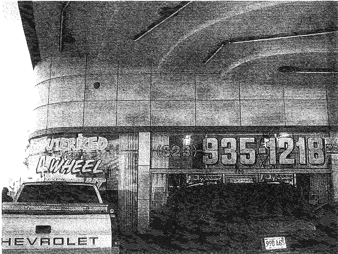
Firestone Tire Building, porcelain wall, 800 S. La Brea Avenue, October 29, 2011 (Photograph by Charles J. Fisher)
