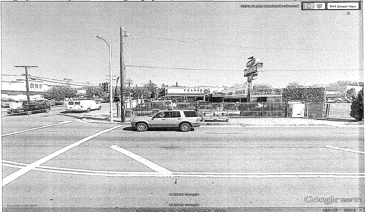
Low-level commercial structures located immediately west of site for proposed 60-foot-tall project.
