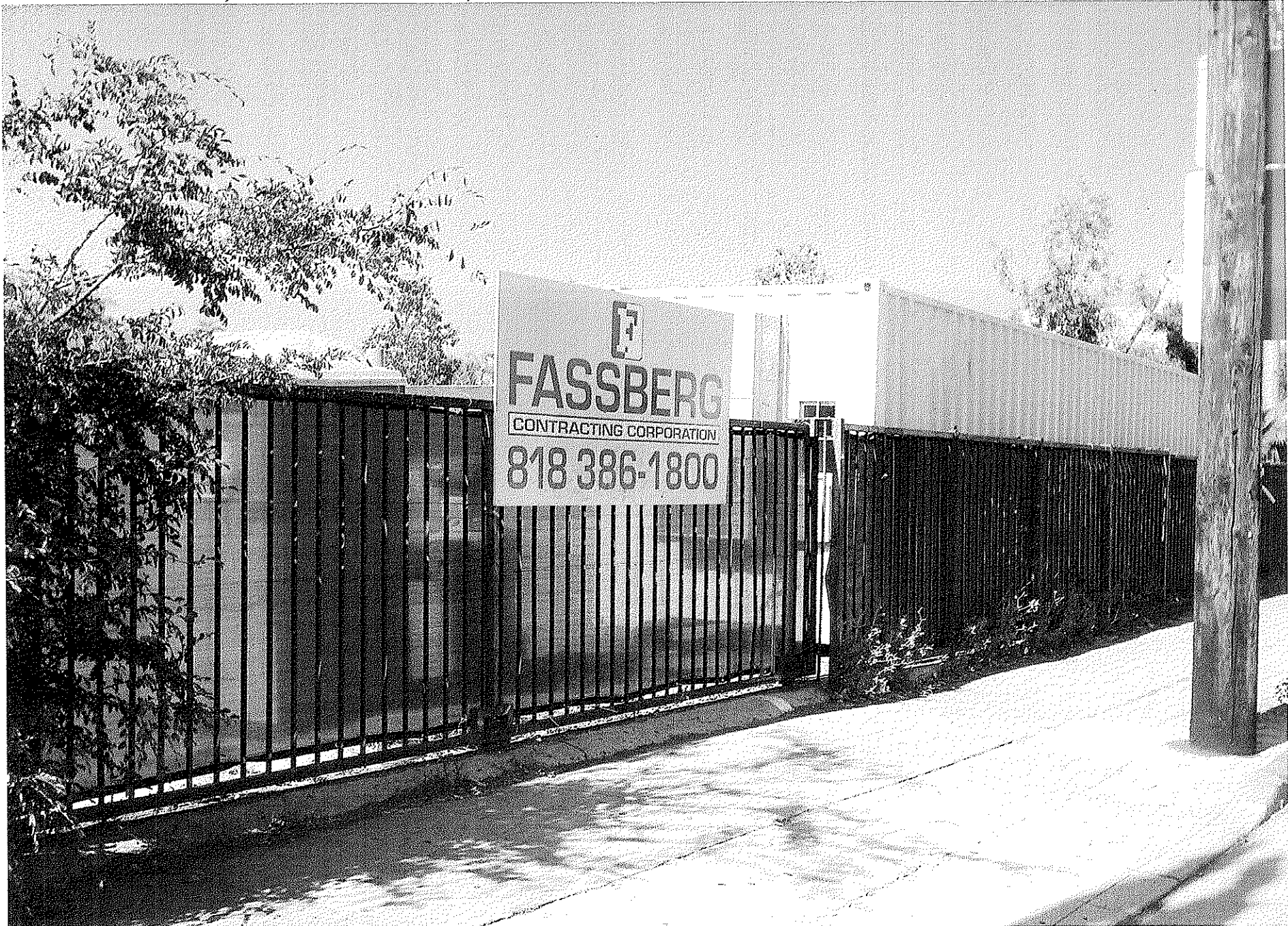
Photo taken June 16, 2013, showing construction office on project site, and perimeter fencing in place, without City approvals.
