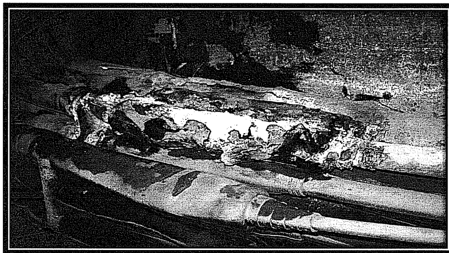
Figure 45: Illustrative of Cable Scheduled for Replacement
