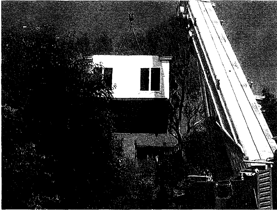
John A. Donnelly House lifted up to foundation in Garvanza, 1121 N. Avenue 64, July 23, 2009 (Photograph by Charles J. Fisher)
