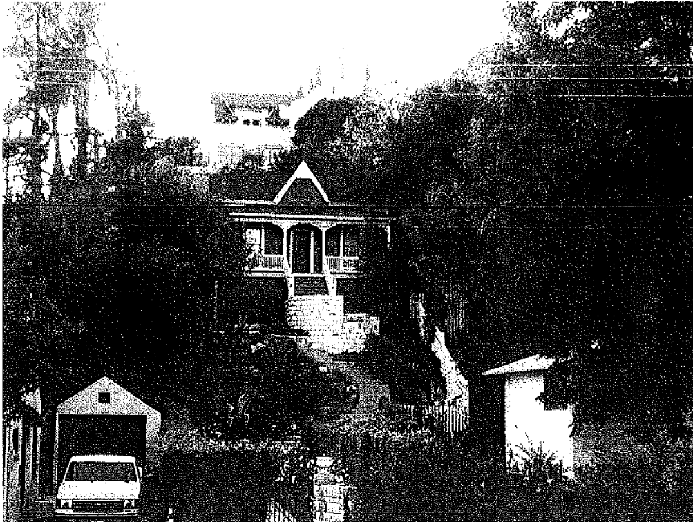
John A. Donnelly House in Garvanza after stairs were oriented back to the front, 1121 N. Avenue 64, October 8, 2012 (Photograph by Charles J. Fisher)
