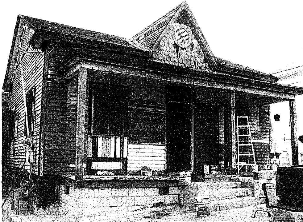
John A. Donnelly House, in Chinatown, 829 W. Bartlett Street, March 2, 2009 (Photograph by Charles J. Fisher)
