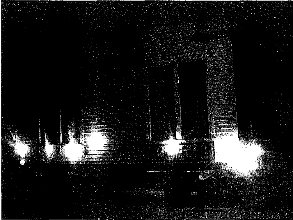
John A. Donnelly House, former East facade with original window openings during move to Garvanza, June 26, 2009 (Photograph by Charles J. Fisher)
