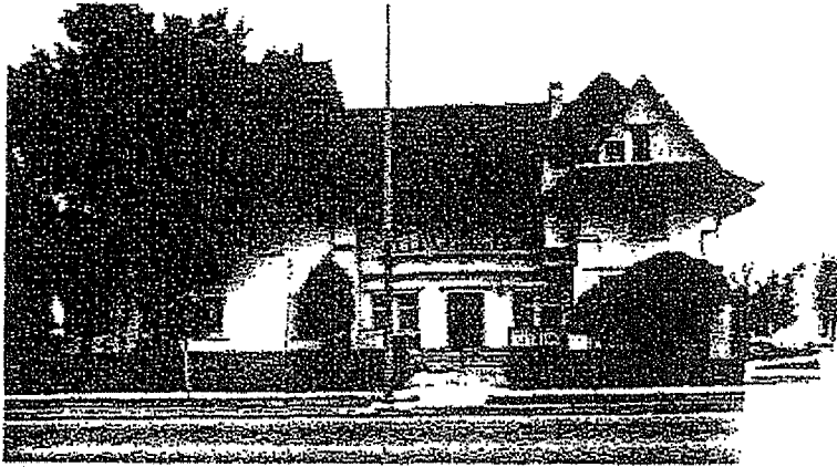
Figure 1: Image of 1342 W Adams Blvd. taken from the North University Park Historic Resources Survey (1983).
