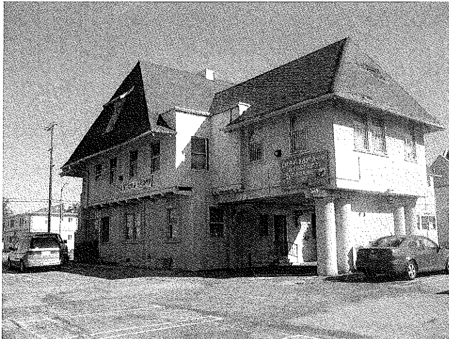
West elevation, viewed from the southwest; south elevation of added porte-cochere and second story chamber.
