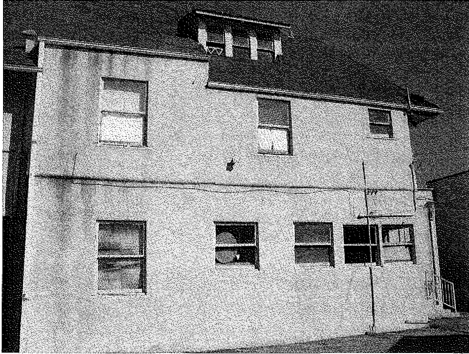
East end of south elevation, view to northeast.
