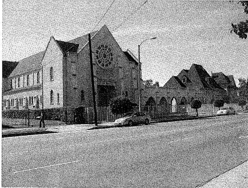
Project viewed to southeast from Roger Williams Baptist Church, to Cloister, to former residence, with east and south additions.
