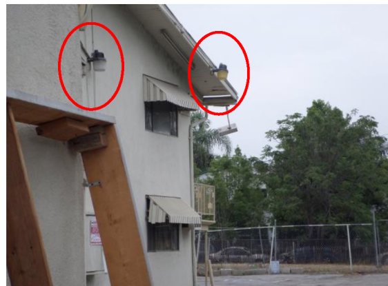
Rear parking area with two exterior lights along the west- facing wall
