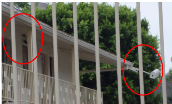
Cameras along stairway in northerly courtyard
