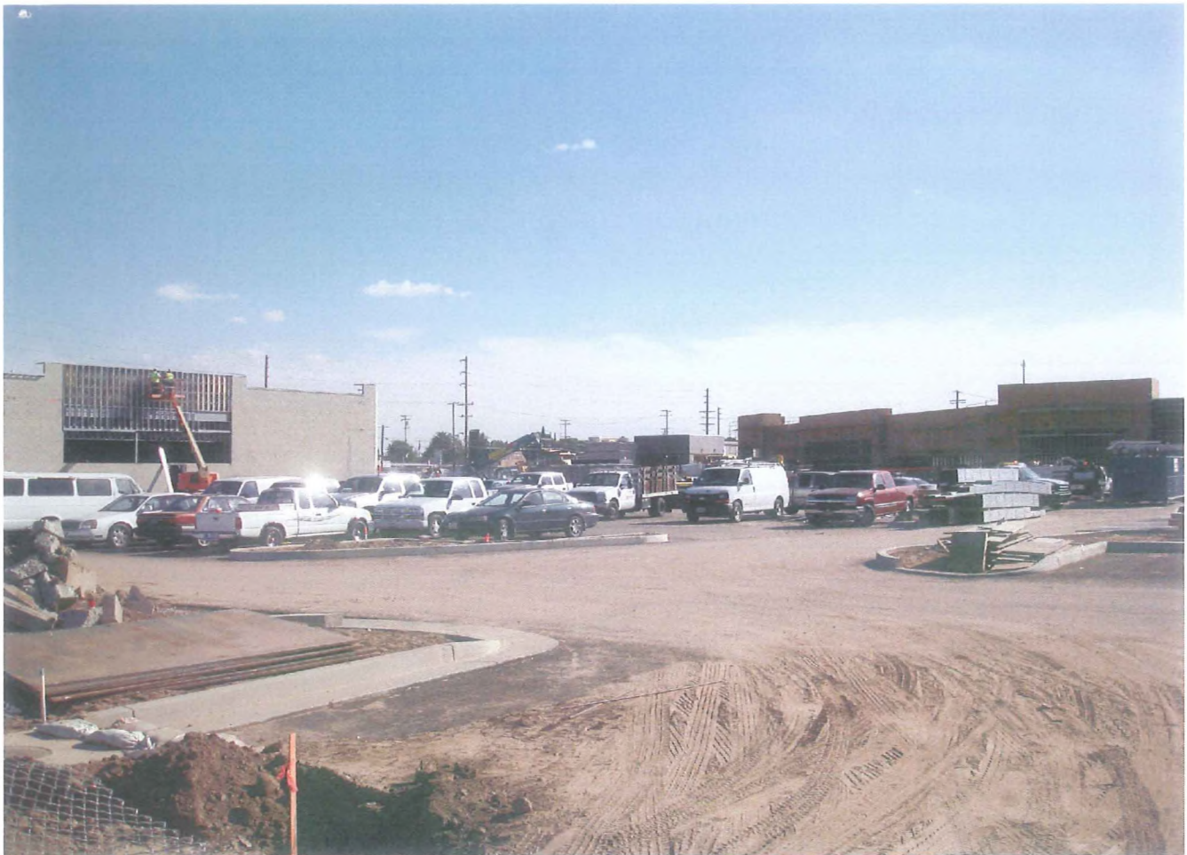
View of new shopping center with CVS Pharmacy building under construction on the left
