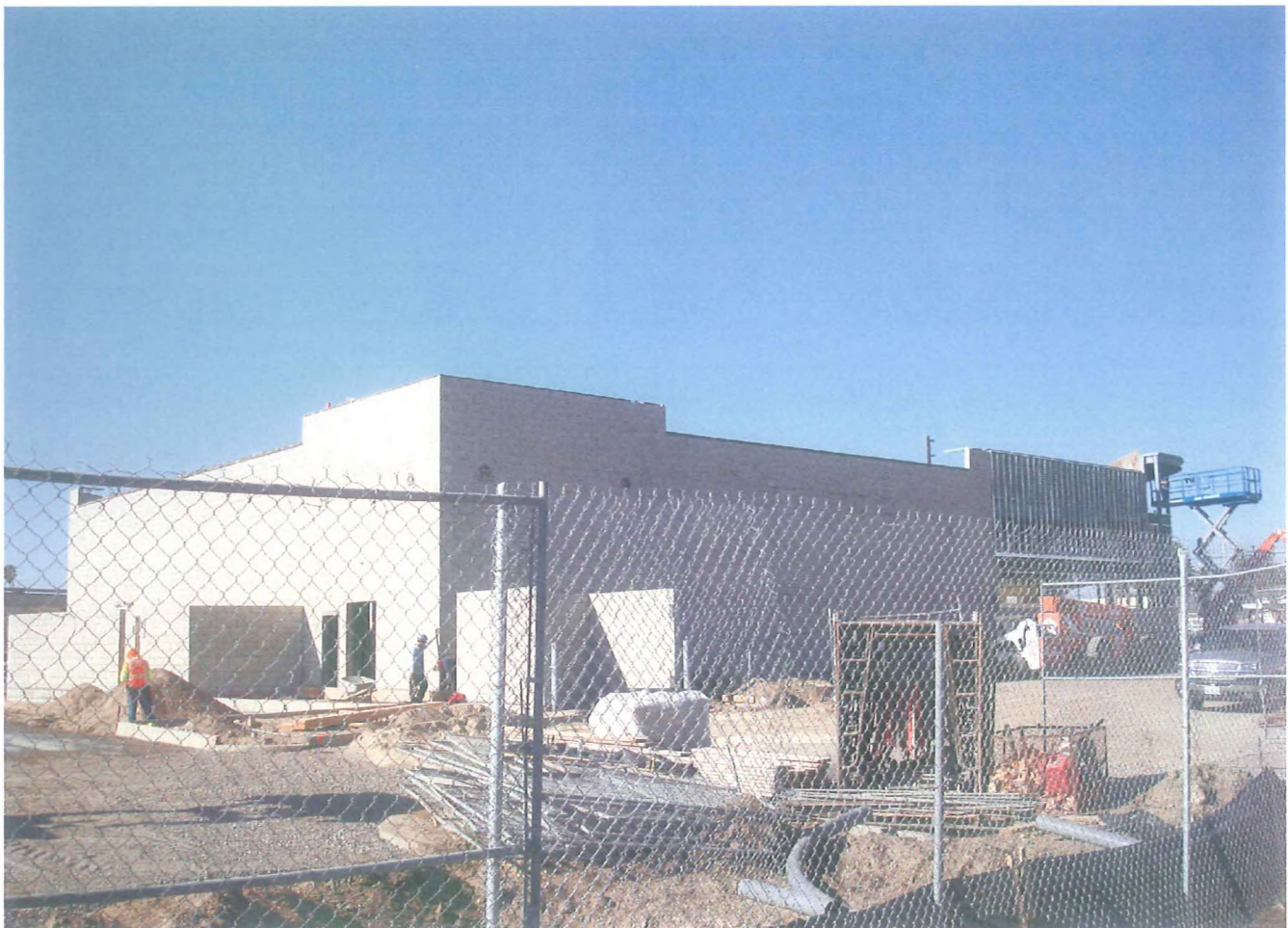
East side of the CVS Pharmacy building taken from driveway off Central Avenue
