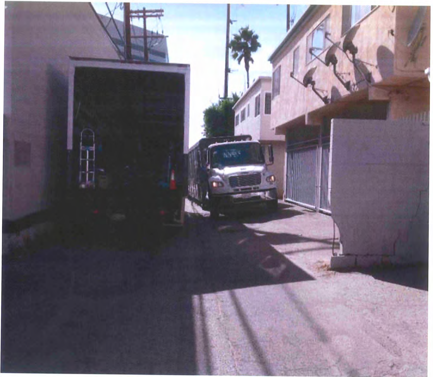
In this photo, note the dent (lower right hand side) in the wall that apparently was made by a vehicle that hit it and tore out a sizeable piece of it and caused a crack in the wall. Also note parked truck on the left and the delivery truck trying to squeeze by.
