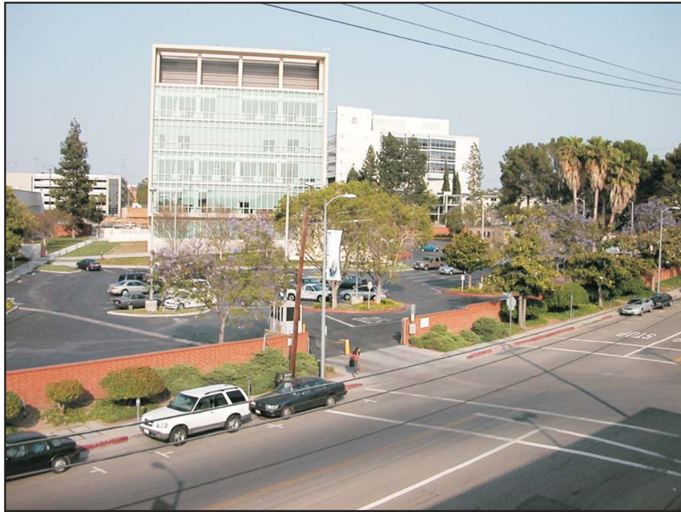
The view eastward from the corner of Biggy Street and Eastlake Avenue shows the new Zilkha Neurogenetics Institute (ZNI) with adjacent surface parking lots that comprise Development Site A.
