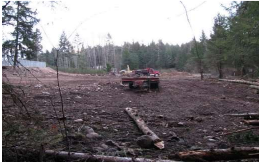
Fig. 4. Photograph: Horkings-Brigham, M. (2015). Unpermitted deforestation and land conversion on 3 acres of hillside in marijuana operations close to a large wetland area outside of Yelm, WA (Thurston County Permitting and Land Use, 2017).
