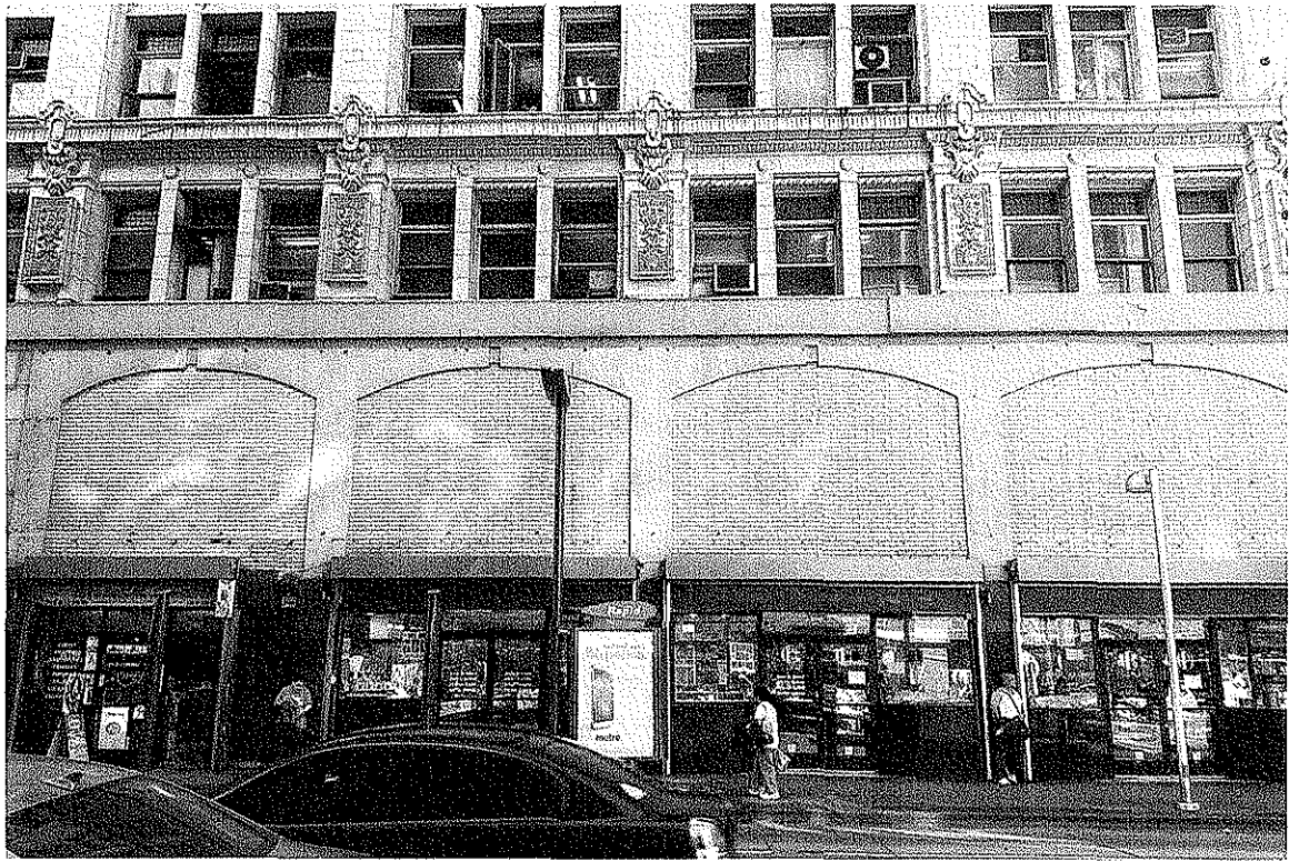
FROM W 6TH ST LOOKING SW (BACK)
