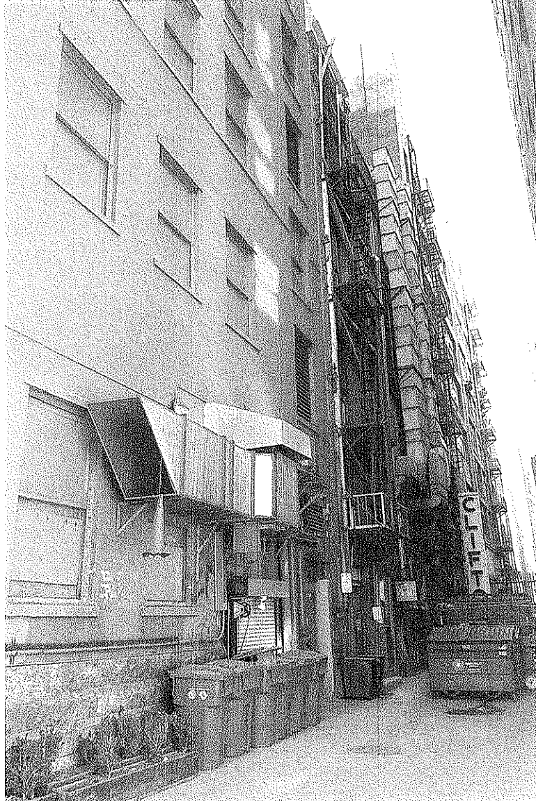
FROM ALLEY LOOKING NW (RIGHT)
