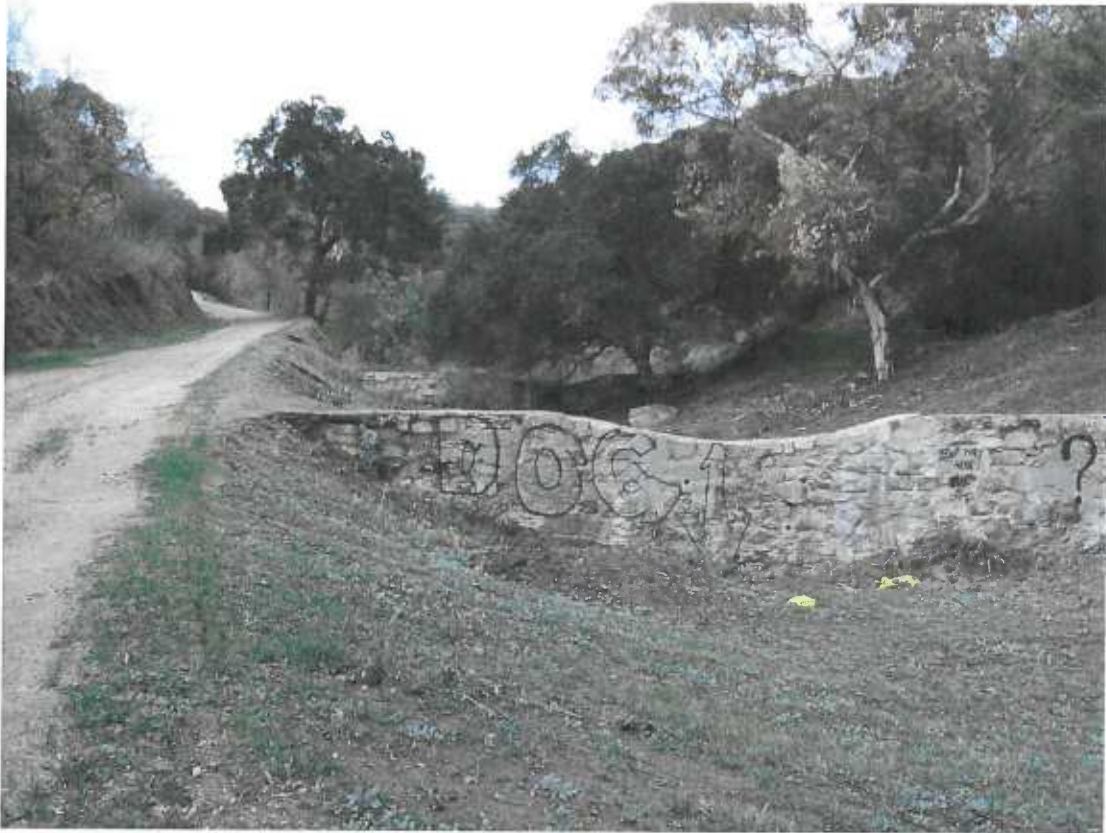
Figure 8. “North Fork” Spring Canyon showing unused check dams.
