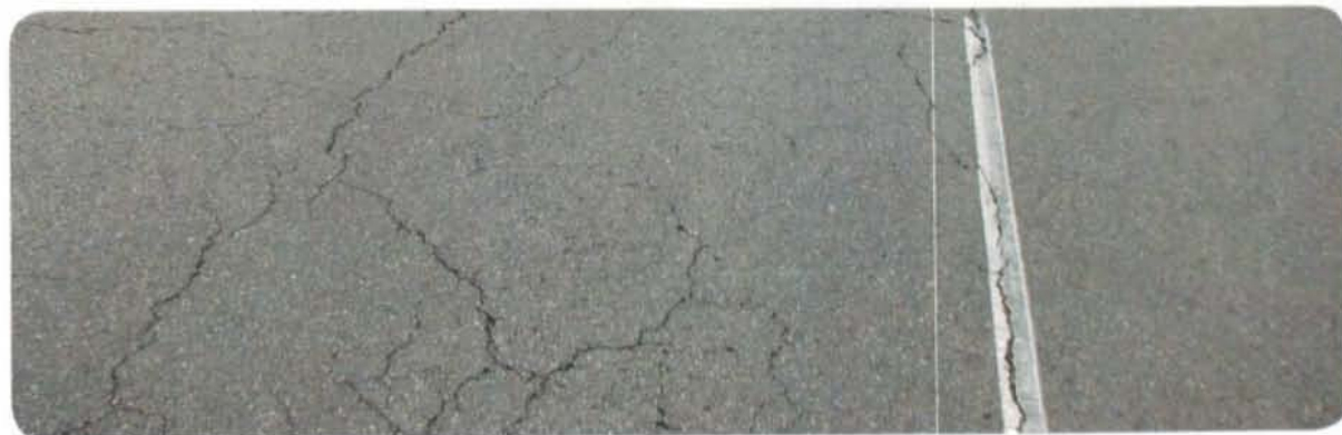
Figueroa & 48th, Pavement Condition Index 57, Grade C-
