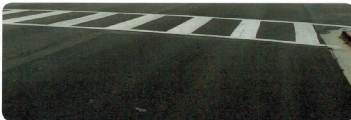
Figueroa - 42nd to 43rd, Pavement Condition 100, Grade A
