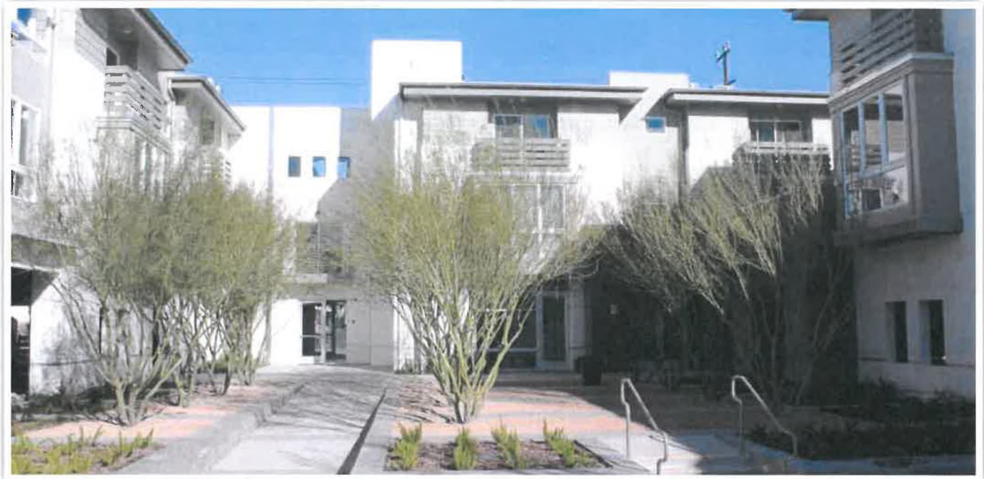
LA Family Housing's Palo Verde Apartments.
