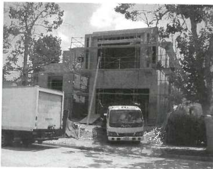
“McMansion” under construction at 808 S. Ridgeley.
